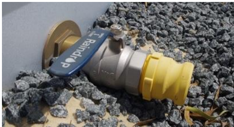
Tank standard camlock fitting
