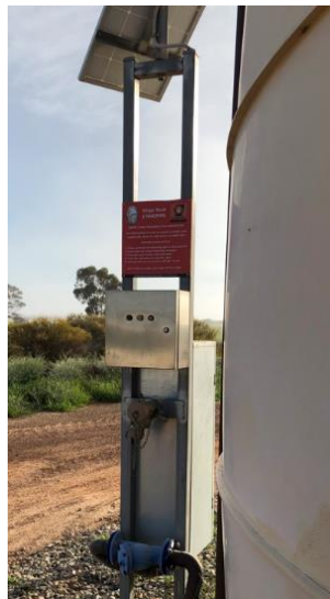
Swipe card standpipe system
