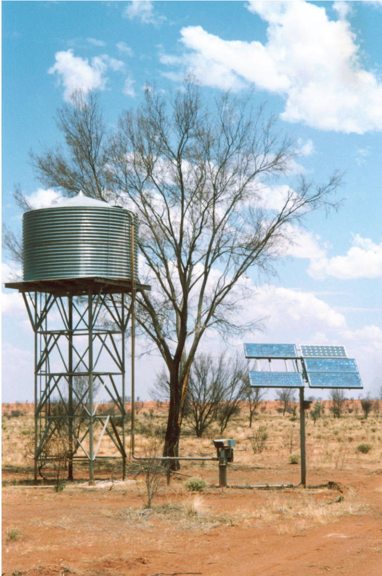
Old orchard water tank and solar pump – not in service
