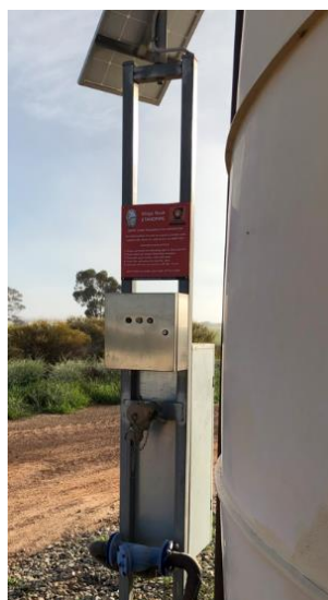
Swipe card standpipe system
