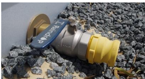
Tank standard camlock fitting
