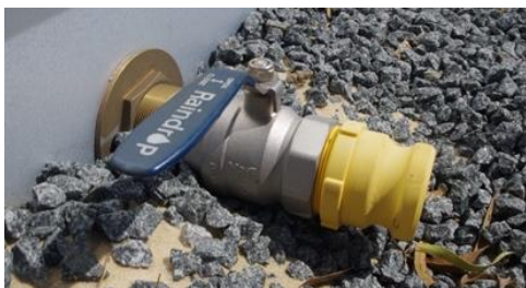
Tank standard camlock fitting
