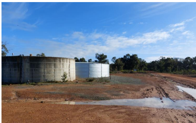
Concrete tanks, 90 kL concrete and 250 kL steel tank on Gnowellan Road (July 2022)
