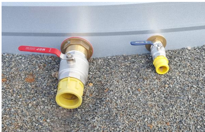
Camlock couplings on 250 kL steel tank
