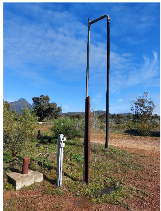
Standpipe with pump switch
