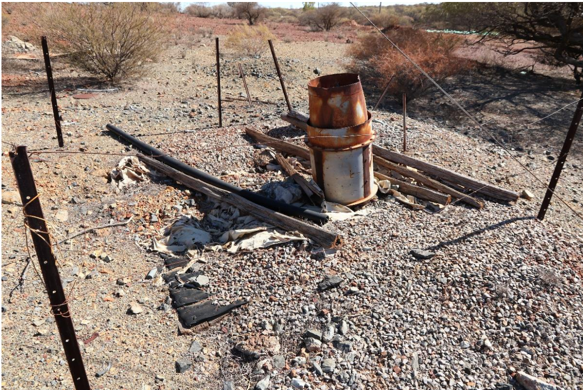
Figure 2: Rose Marie Shaft with dilapidated fan positioned over shaft
