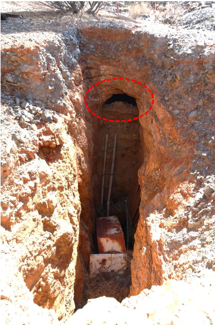
Figure 3: Open stope north of Main Shaft, facing northeast, also showing (red dashes) secondary void in the northern face of the stope. Debris can be seen blocking the stope at about 3 m depth.
