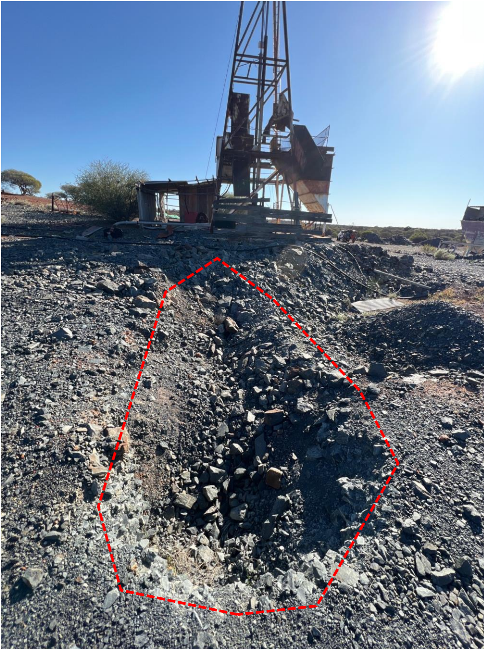
Figure 4: Area of subsidence within stockpiles mine waste, southwest of Main Shaft, looking northeast
