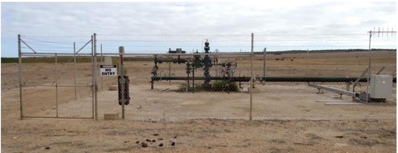
**Figure 5:** The principal component of a petroleum production well that is visible on the surface is the Christmas tree, an assembly of valves and pipework fitted to the wellhead to control the flow of oil or gas production from the well to a pipeline or a production facility
