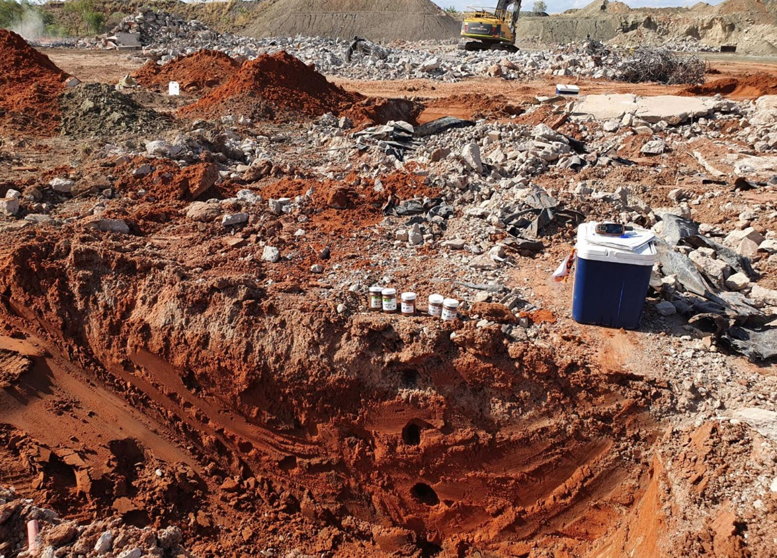
**Sampling the soil profile underneath what was the E9 fuel farm to determine the presence of hydrocarbons.**
