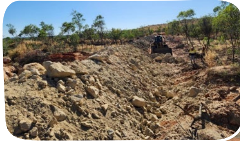
Safety bunds established around the pit voids.
