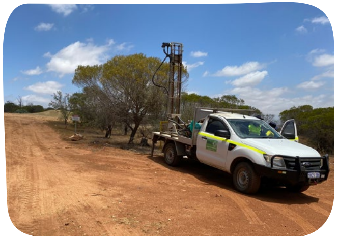
Auger rig at Commonage during geotechnical assessments.
