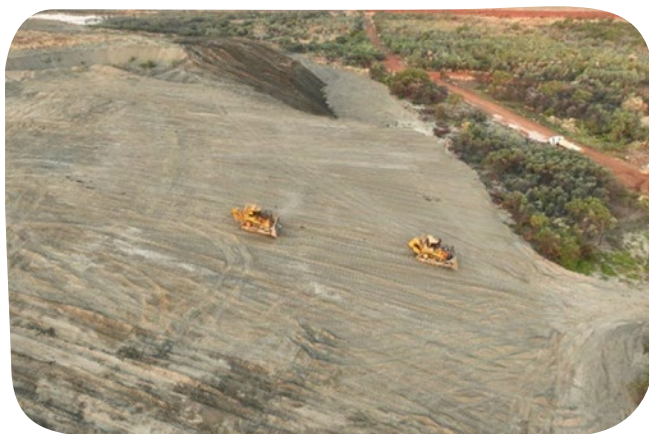
E9 Lights Stockpile showing some of the before profile and during works.
