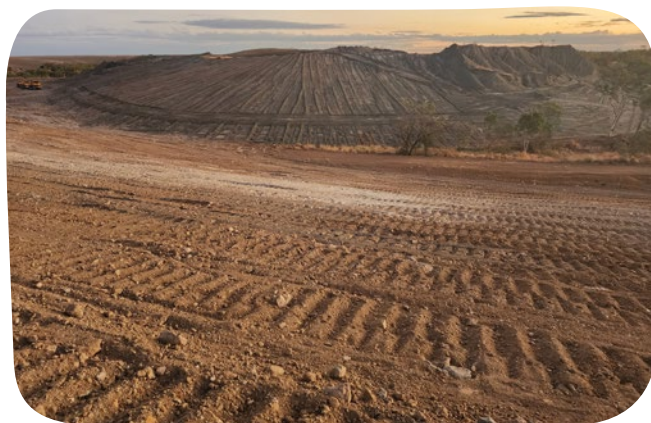
E9 ROM and Noise Bund landforms – works in progress.
