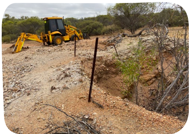
Geotechnical assessment test pits between abandoned shafts.
