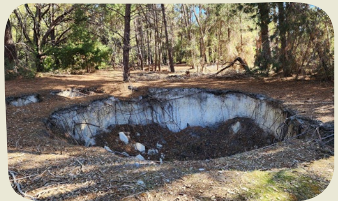
Neath/Cardiff Colliery recent subsidence indications.
