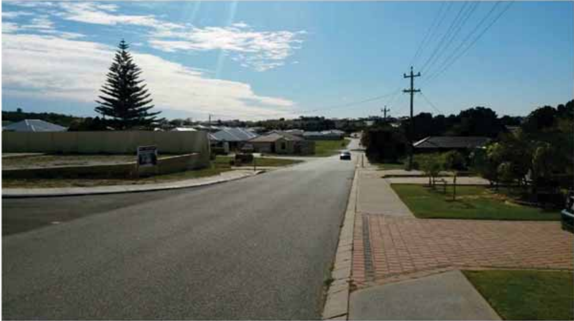
Figure 4: Northbound view along Watson Road in the vicinity of the East-West road intersection
