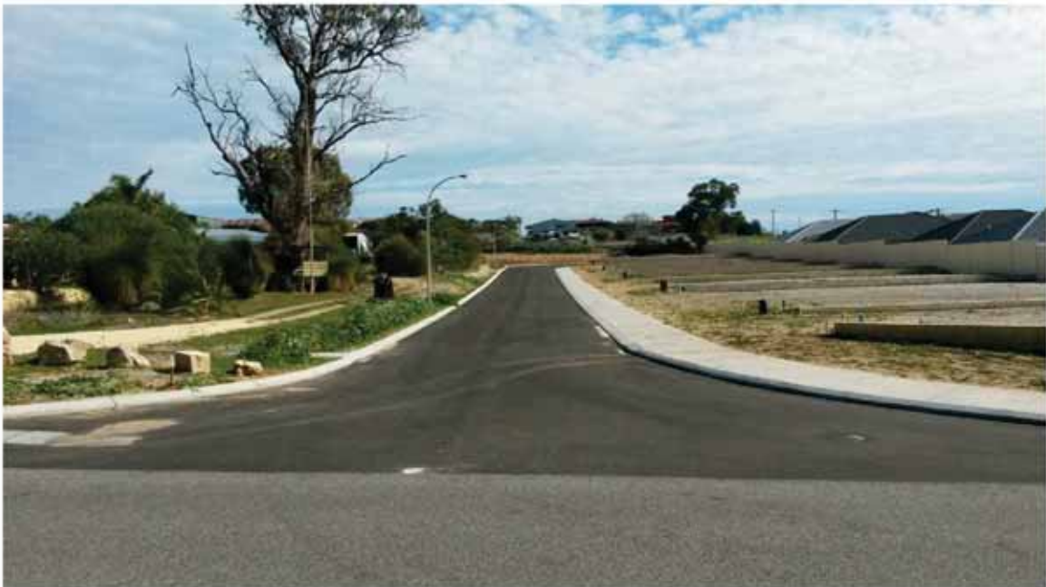
Figure 5: Westbound view along East-West road from the Watson Road intersection
