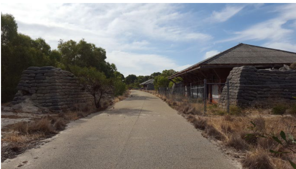
Figure 26. Remaining munition magazines, Woodman Point
