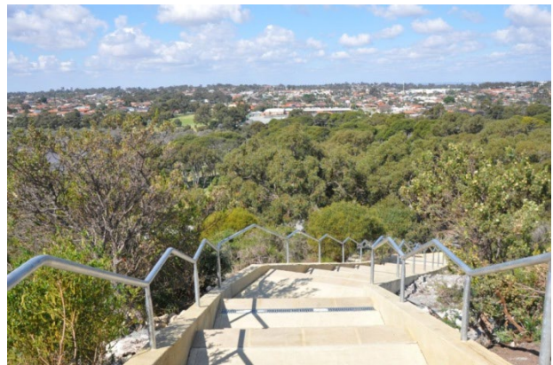
Figure 58. Manning Park stairs
