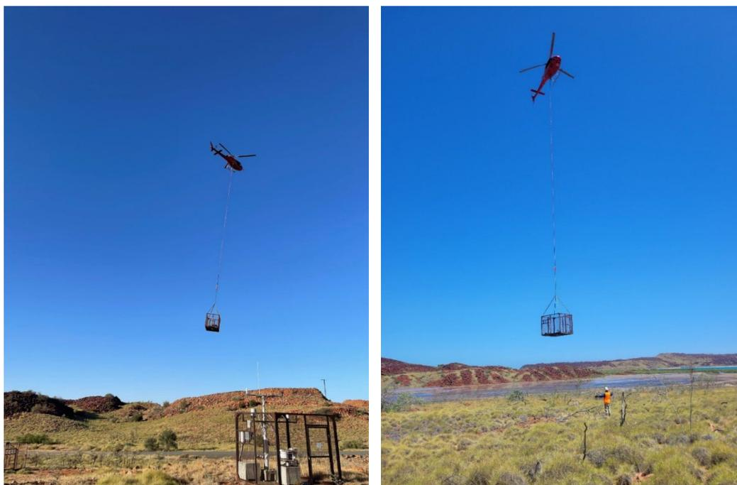
*Helicopter installation of passive Air Quality Monitoring cages on island sites*
