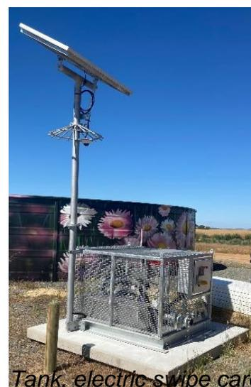
*Tank, electric swipe card and pump for bore*
