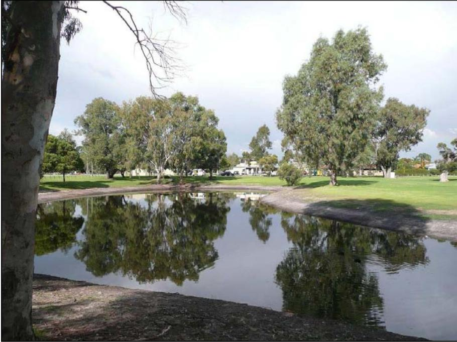
**Figure 3-5:** *Constructed lake in the catchment's north-east which is effectively a large drainage sump in a low-lying region of a park*
