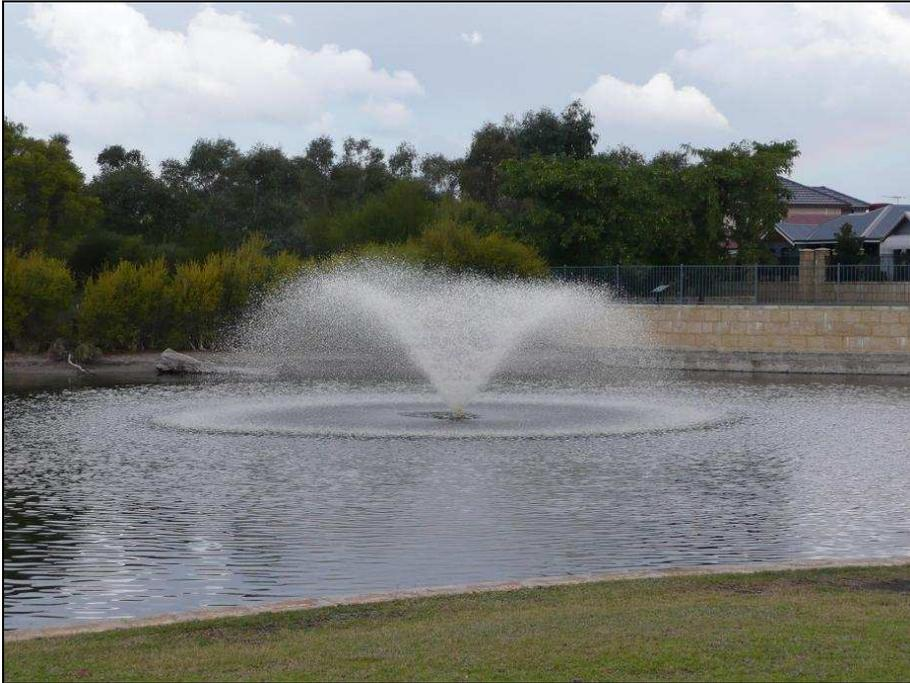
**Figure 3-3:** *Constructed lake in public open space, with features including concrete-lined walls and aeration fountain*
