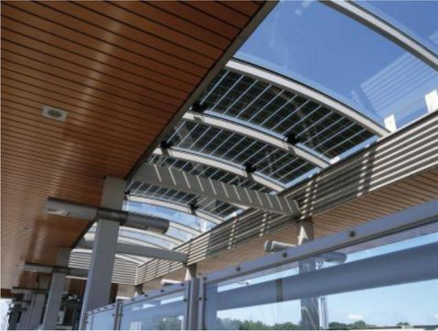
Image 43: Solar Panels Integrated into Awnings
