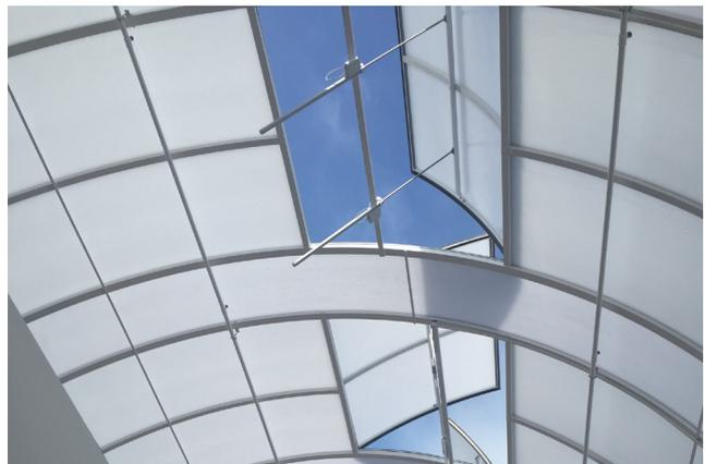
Image 14: Barrel Vault Roof Lights
