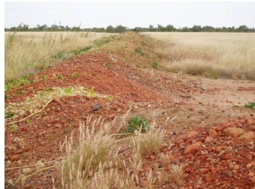
**Figure 11 - levee bank on southern perimeter of living area**
