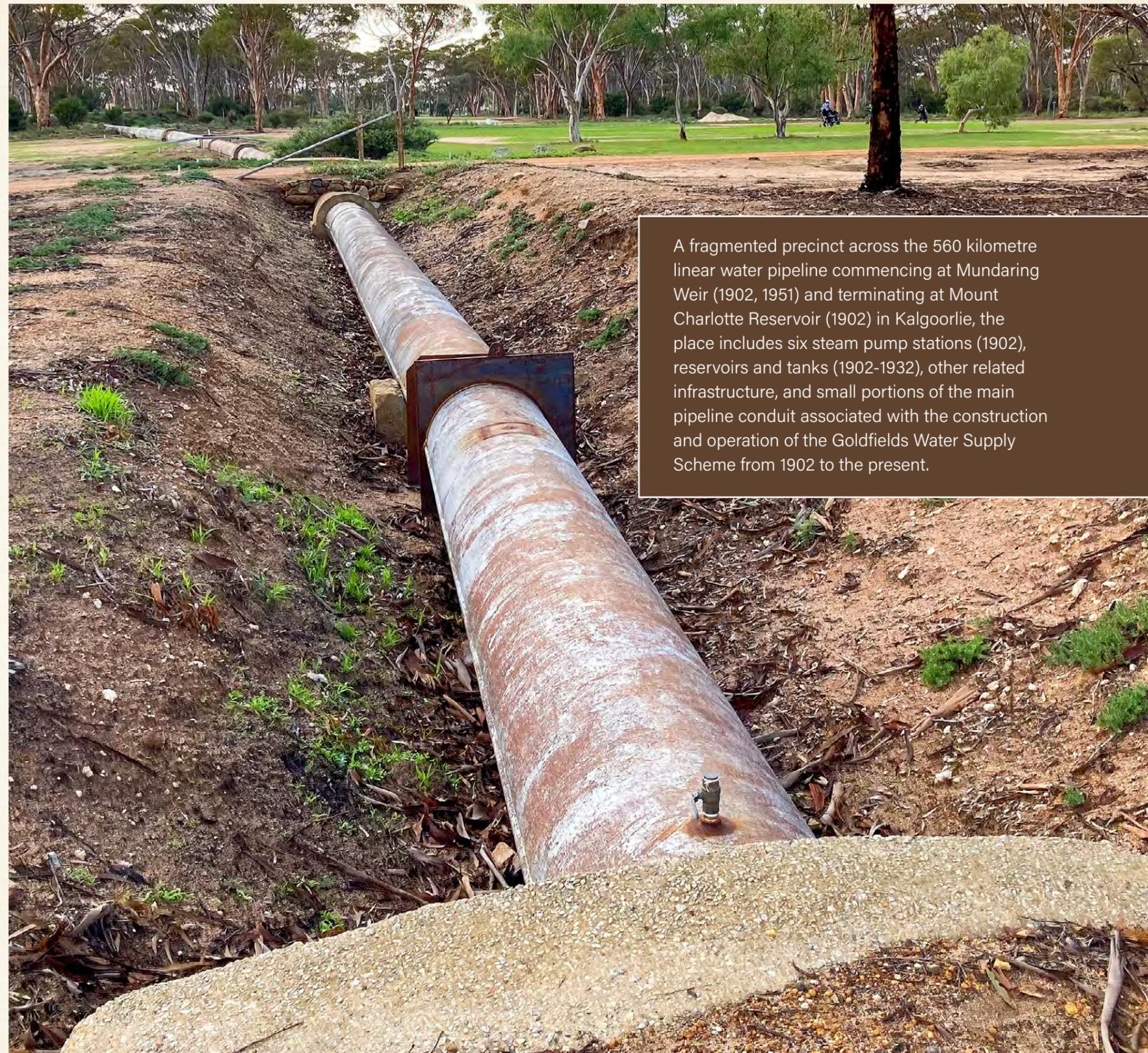
A fragmented precinct across the 560 kilometre linear water pipeline commencing at Mundaring Weir (1902, 1951) and terminating at Mount Charlotte Reservoir (1902) in Kalgoorlie, the place includes six steam pump stations (1902), reservoirs and tanks (1902-1932), other related infrastructure, and small portions of the main pipeline conduit associated with the construction and operation of the Goldfields Water Supply Scheme from 1902 to the present.
