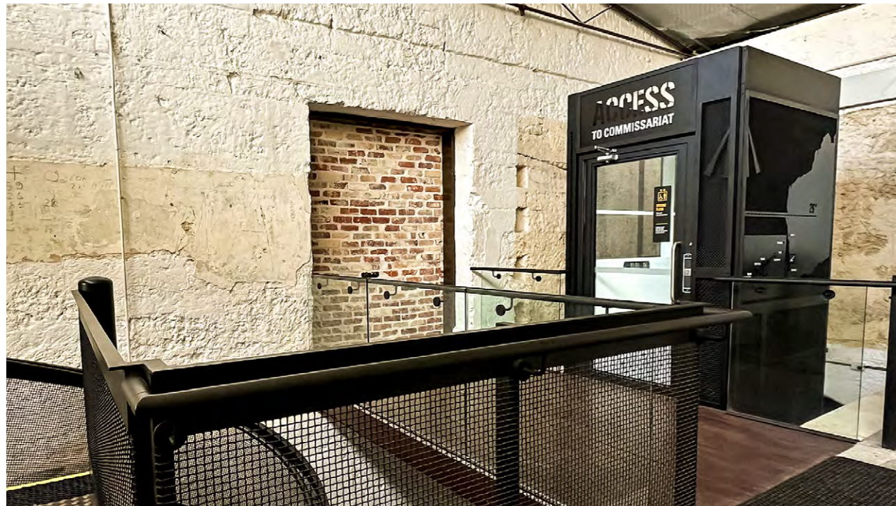
Universal access lift to the Commissariat, Fremantle Prison.
