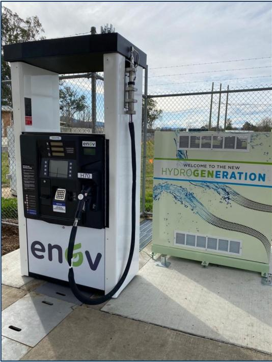
**Figure 3.18** Vehicle Hydrogen Refuelling Skid
