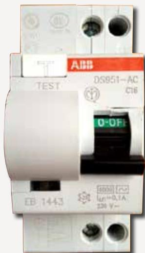
If the lever doesn't flip downwards or you notice any other problem with your RCD you need to contact Housing Direct on **1300 137 677**.
