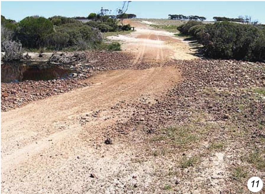
It is possible that a ford crossing will slightly increase water depth upstream. It is important that the bank is protected where the access track enters the floodway to reduce the risk of high flows eroding these points. Inadequate placement and continuity of bed armouring material along the upstream and downstream edges of a crossing is common and creates weaknesses in the overall structure.
