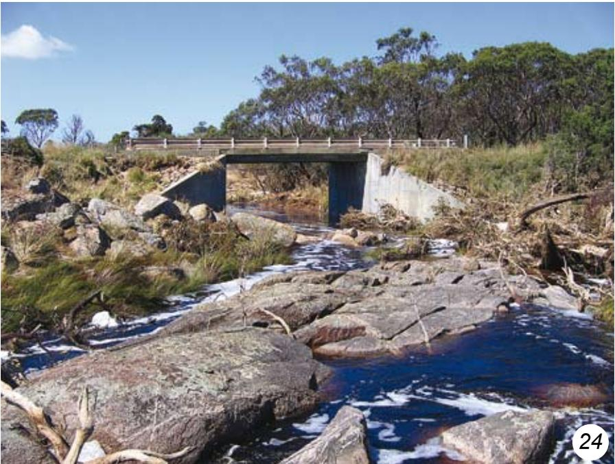
bridge design. The height of the bridge maintains the cross-sectional area of the channel and concrete supports are winged, which assists in guiding the flow under the bridge. The winged supports also help armour the banks.
