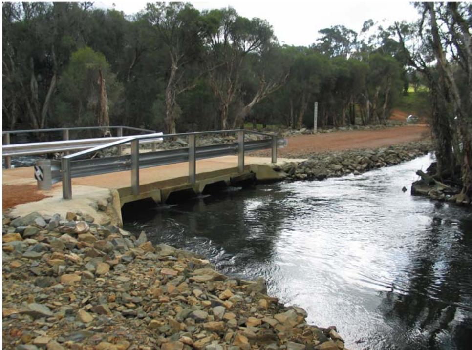
*Figure 10.* Box culverts installed at William Street crossing to facilitate fish passage on Hotham River, July 2005.
