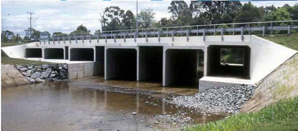
*Figure 6.* A multi-celled box culvert crossing to allow movement of aquatic and terrestrial fauna beneath a road crossing (Fairfull and Witheridge, 2003)
