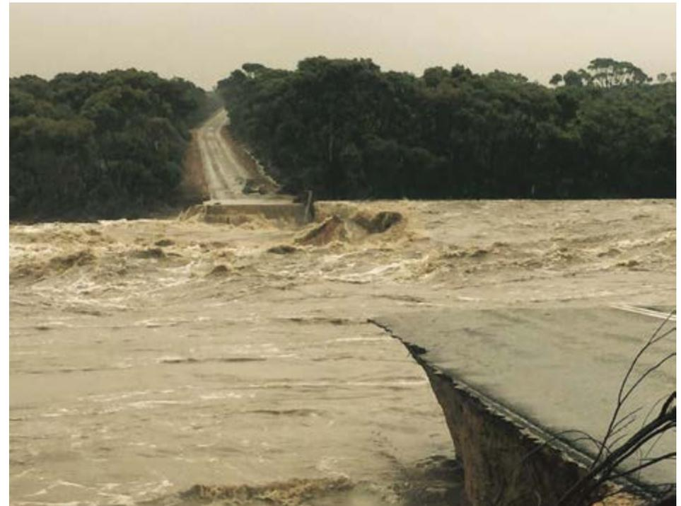
**Figure 3. Flood damage to Phillips River Bridge near Ravensthorpe**
