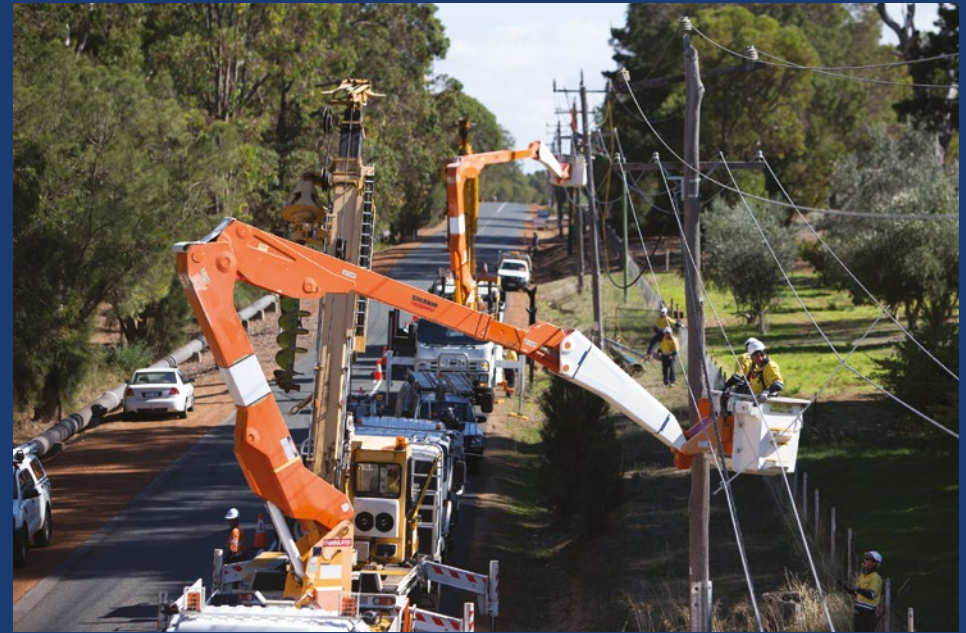
Figure 17. Western Power crews working in Lesmurdie
