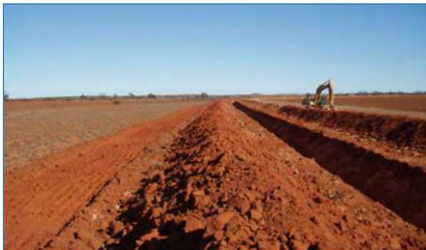
Plate 1: Construction of arterial drain showing central channel, levee banks and surface channel (YYCMG 2010)
