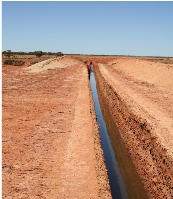
Figure 9 The rock-sawn drain section
