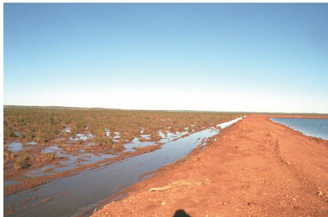
Figure 48 Leakage outside the SE basin wall
