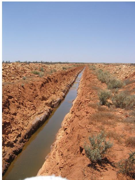
Figure 7 Soil profile typical of the Morawa drain showing loamy topsoil over cemented subsoil
