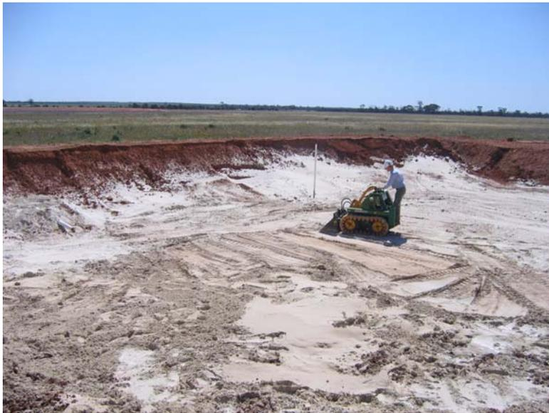
Figure 27 Levelling the lime-sand bed in the floor of the pilot evaporation basin
