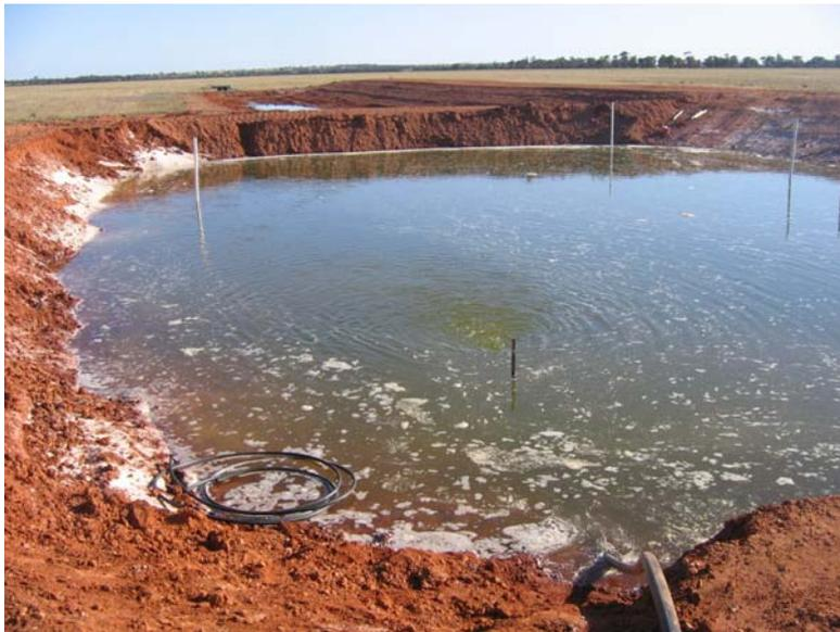
*Figure 28 Pilot lime-sand basin nearing the point of maximum filling (Batch 1)*
