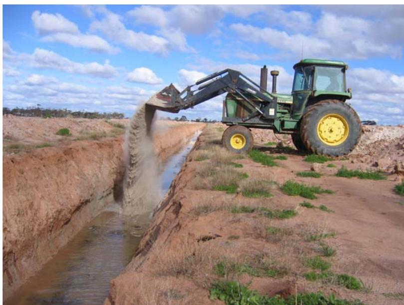
*Figure 13 Loading lime-sand into a drain using a front-end loader: note the opening of the levee banks to allow access*
