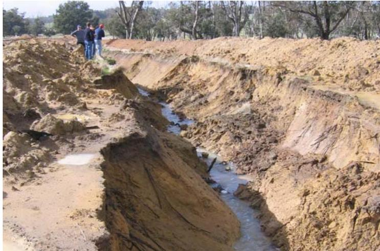
Figure 7 Drain slumping
