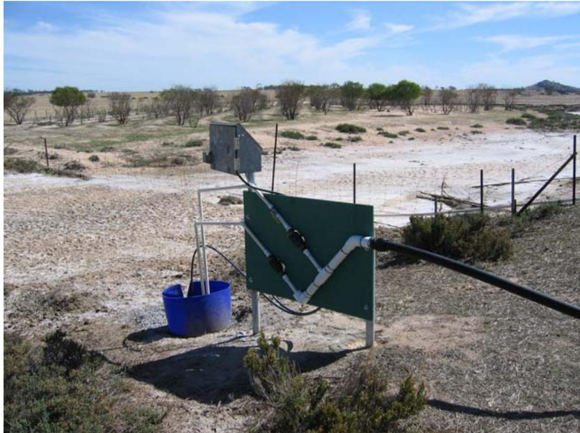
*Photo 2 The flow meter measuring groundwater discharge from the production bore to the creek line*
