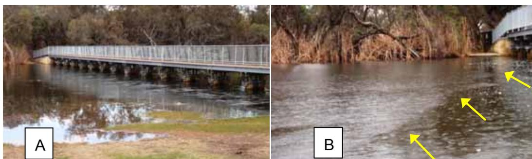
Figure 18 Overtopping of the KSW: illustrating flooding of upstream banks (A) and the mixing line of saline and fresh water (B)
