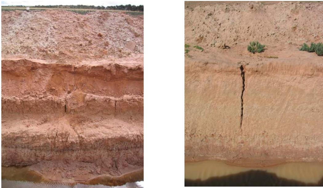
Figure 18 Eroded soil from the levee bank is easily transported across the narrow berm into the drain channel
