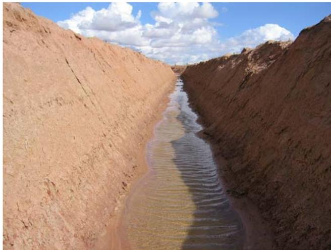
Figure 16 A section of treatment 1 channel with limited erosion at the 3rd survey
