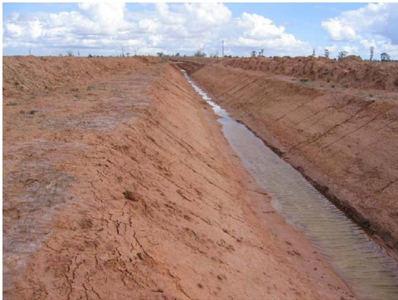
*Figure 7 Treatment 3 (foreground) changing to treatment 2 (background) with the 4-m wide berm on the left side of the channel*
