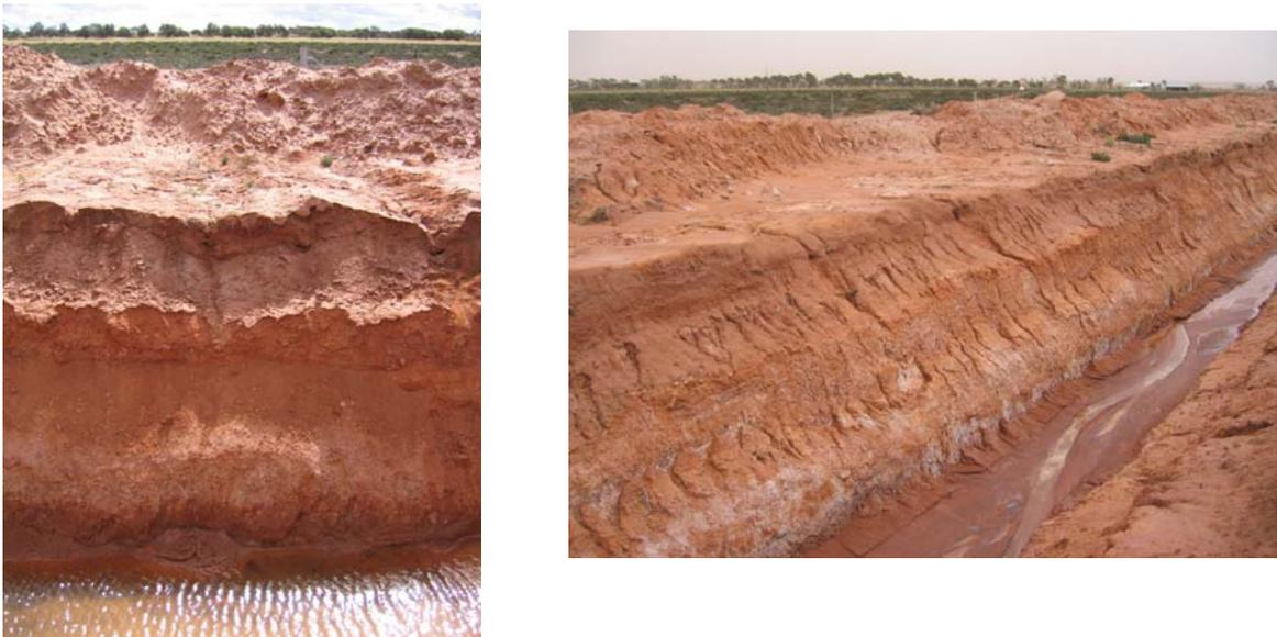
*Figure 14 The step batter breaking down but holding the eroded material on the benches*
