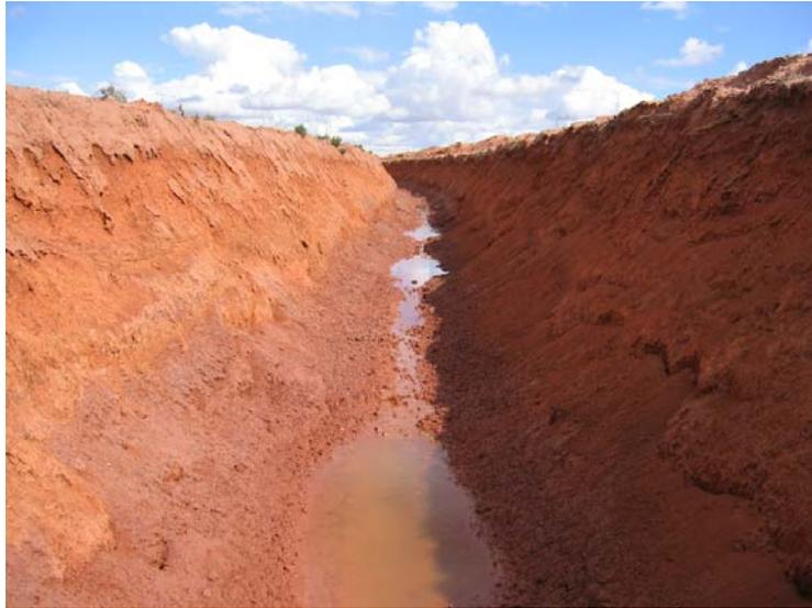
Figure 19 The crumbling batters of treatment 1 in replicate 2
