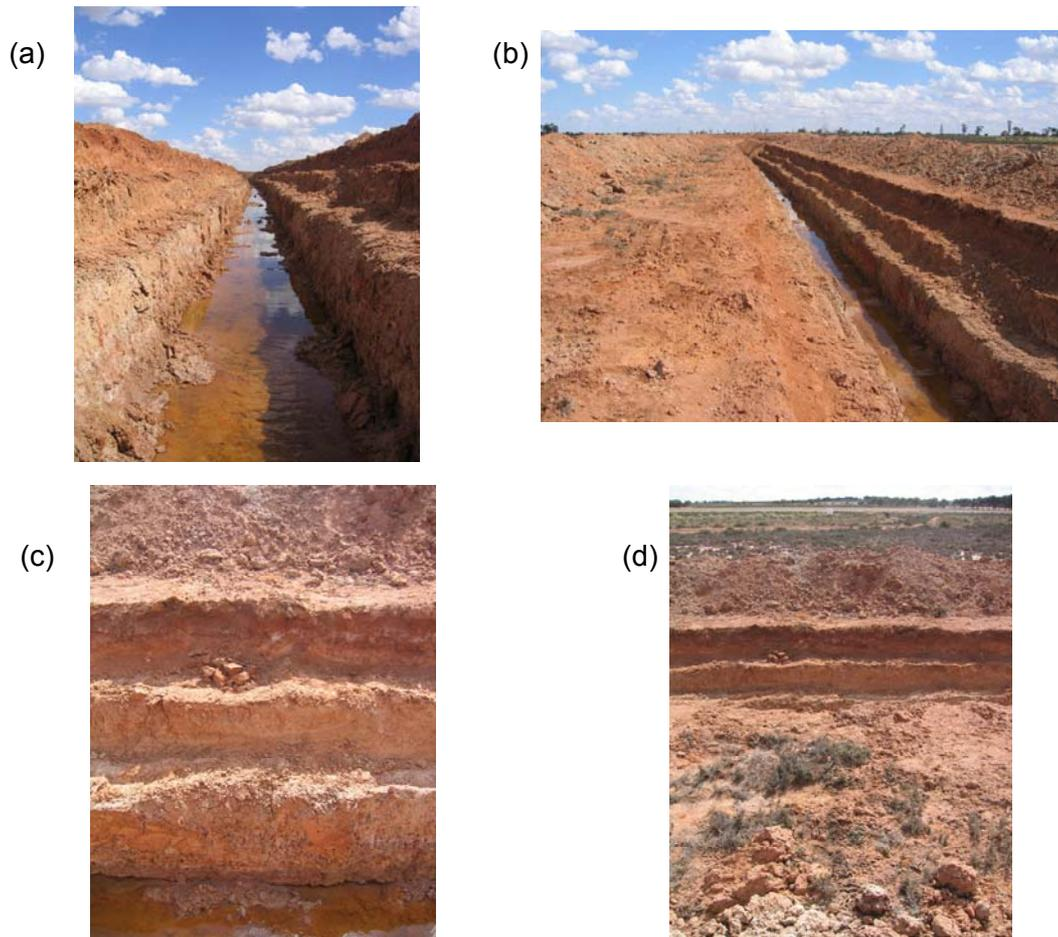
*Figure 9 The photo monitoring set (a) inside channel showing sediment on floor (b) channel overview showing batter condition and berms (c) perpendicular close-up of batter on narrow berm side (d) wide perpendicular view showing both berms of step batter (treatment 2) in replicate 1*
