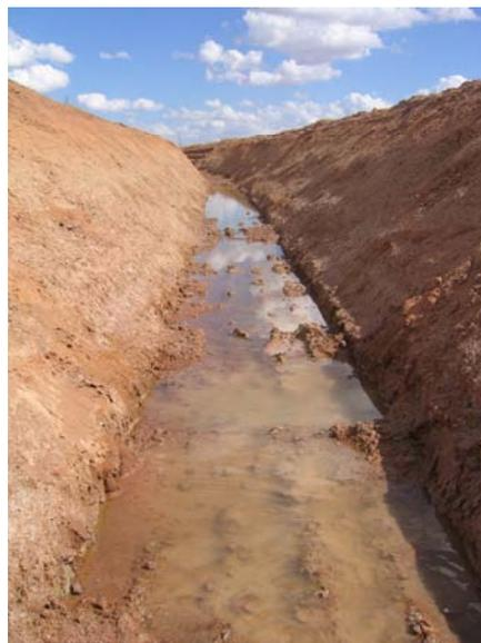
*Figure 15 This section of treatment 3 channel has remained very stable throughout the trial*
