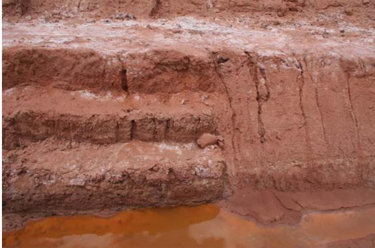
*Figure 4 Sheet, rill and tunnel erosion were visible on all of the drain batters*
