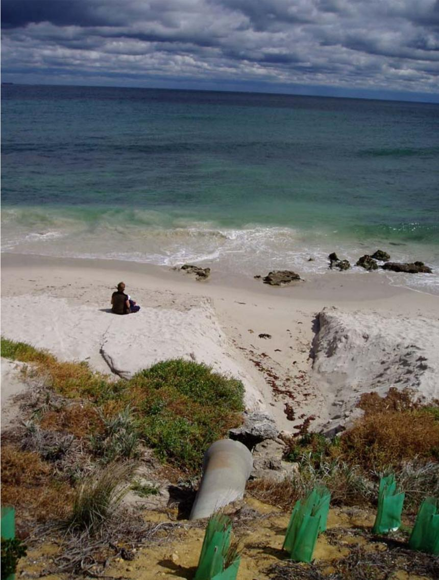
**Drain (NSTO3) at Sorrento Beach showing channel formed by flowing stormwater. Photograph by Helen Astill.**
