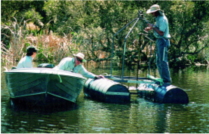
Figure 4: BOC Gases contractors installing dissolved oxygen probes for the automatic control system
