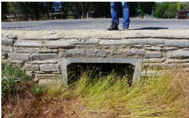
Figure E-13: Bridge B7, Rowley Road, Birriga Main Drain
