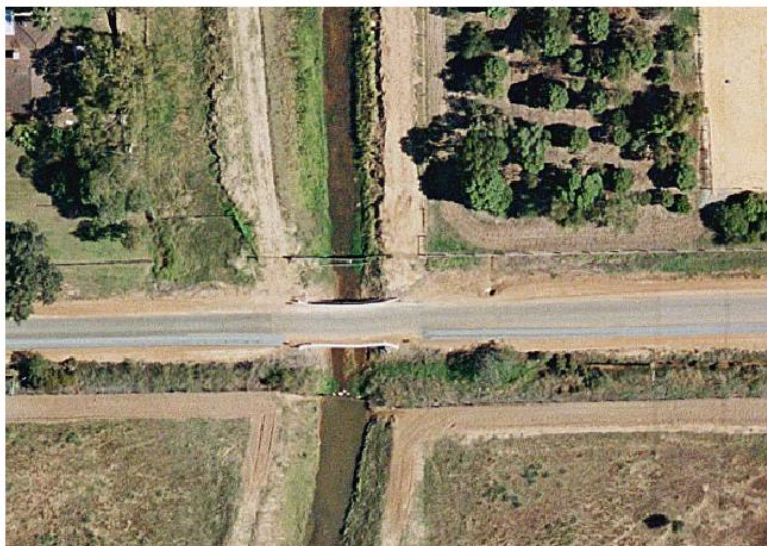
Figure E-5: Bridge O5, DZ013628, Oaklands Main Drain, Gossage Road
