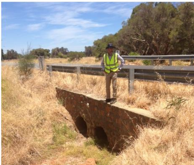
Figure E-11: Bridge B5, Kargotich Road, Birriga Main Drain
