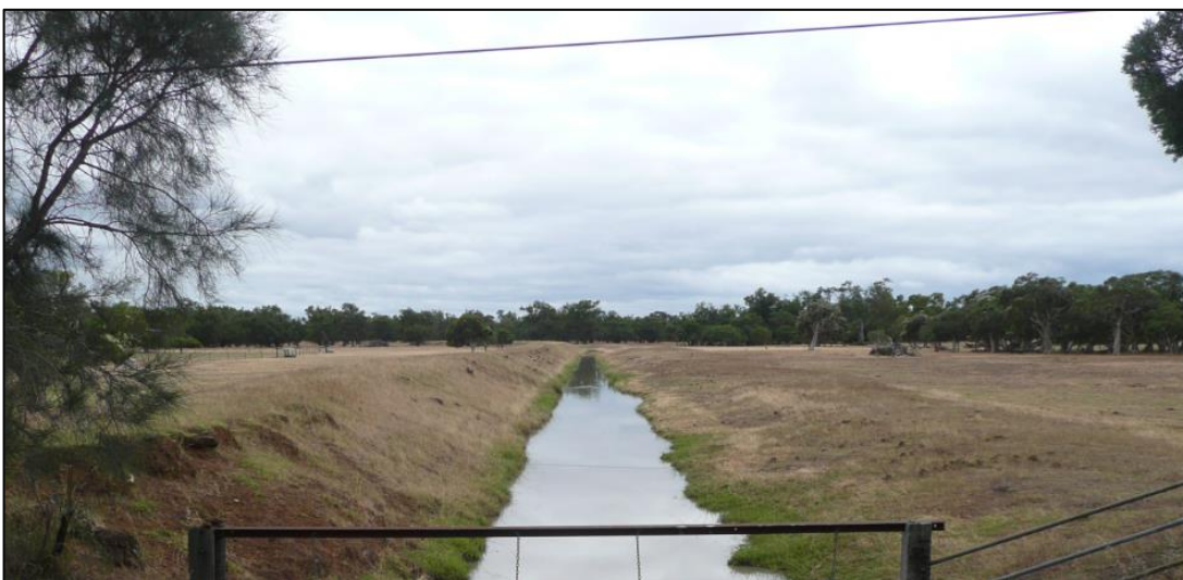
Figure 2-4: Oaklands Drain upstream of Leipold Road (Photo C)
