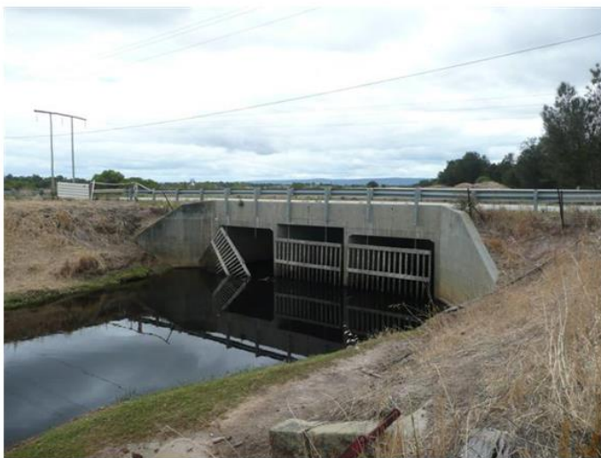
Figure E-7: Bridge B1, DZ014325, Birrega Main Drain, King Road
