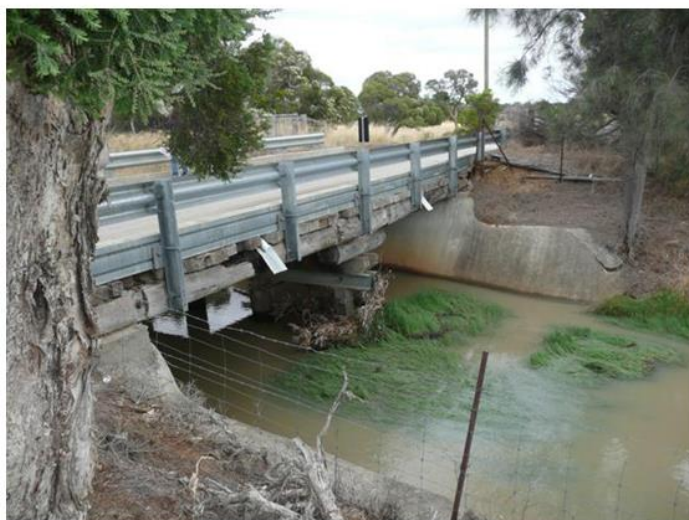
Figure E-3: Bridge O3, DZ013626, Oaklands Main Drain, Leipold Road
