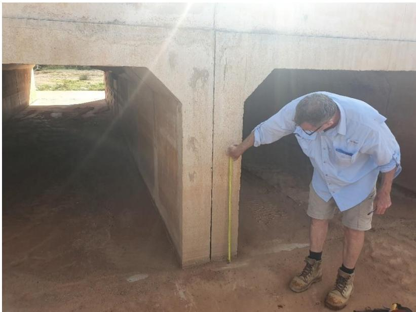
*Figure 17 Measuring up from ground to flood mark (downstream side of culverts at Six Mile Creek crossing of North West Coastal Highway)*
