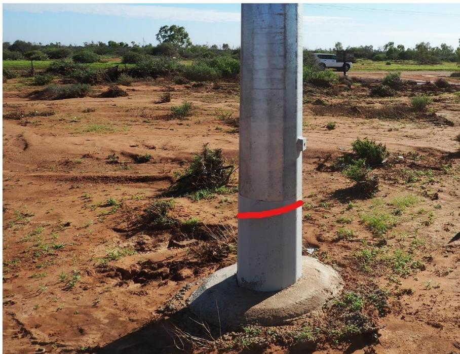
*Figure 18 Flood mark on power-pole (difference in upstream [right] and downstream level [left] has been highlighted)*
