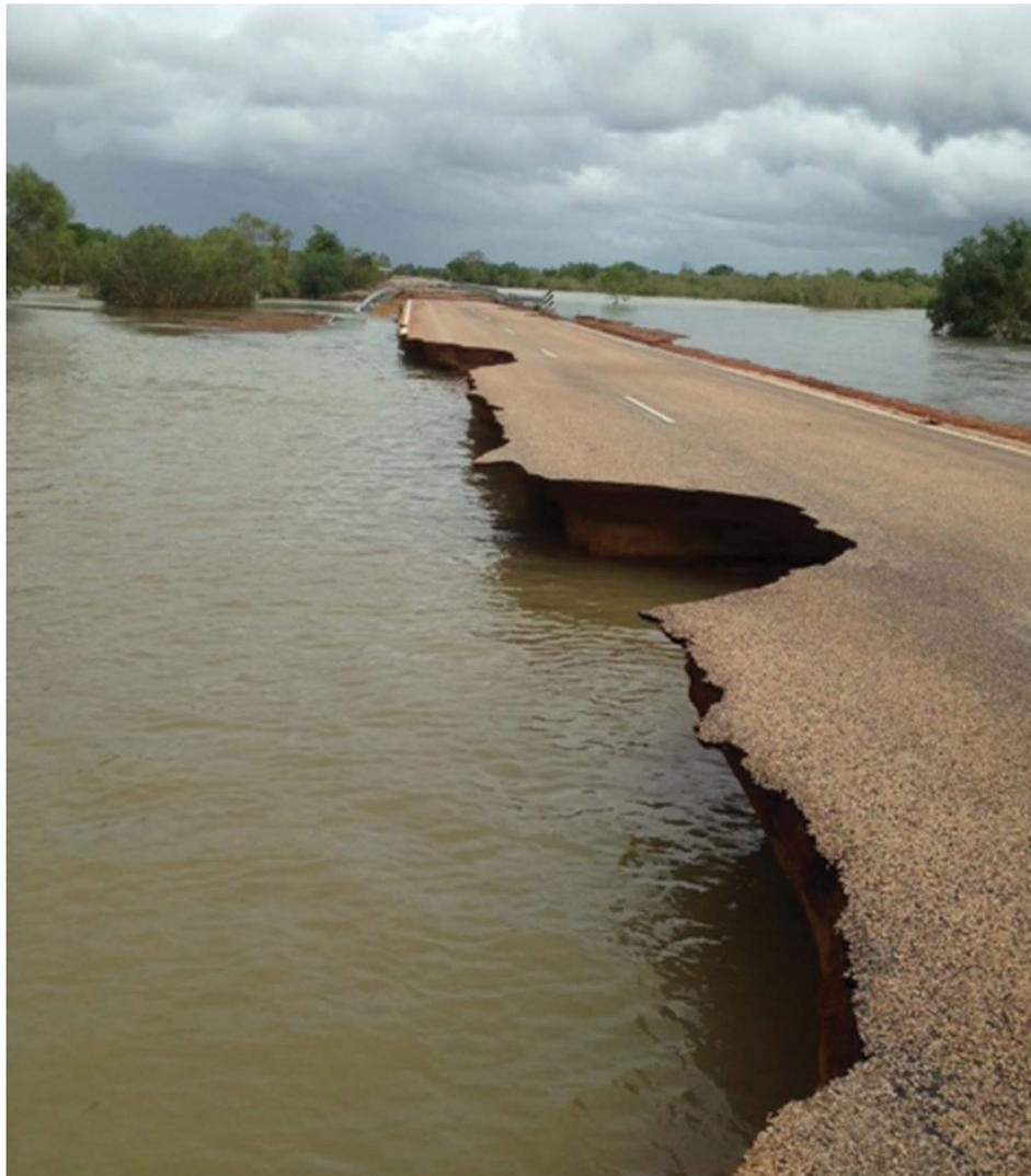
Figure 36. Flood damage near the Logue River bridge in the Kimberley.
