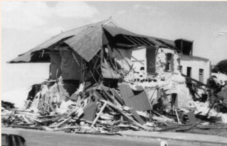
Figure 7. The Meckering Hotel was destroyed by the 1968 earthquake. Source: C. Wadley – The Big Camera
