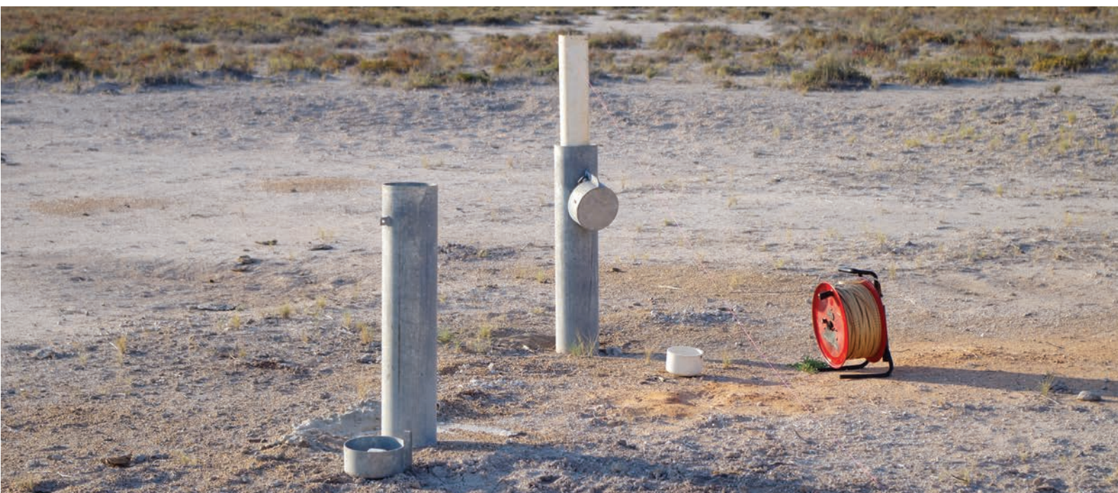
Groundwater investigation bores within the groundwater monitoring network
