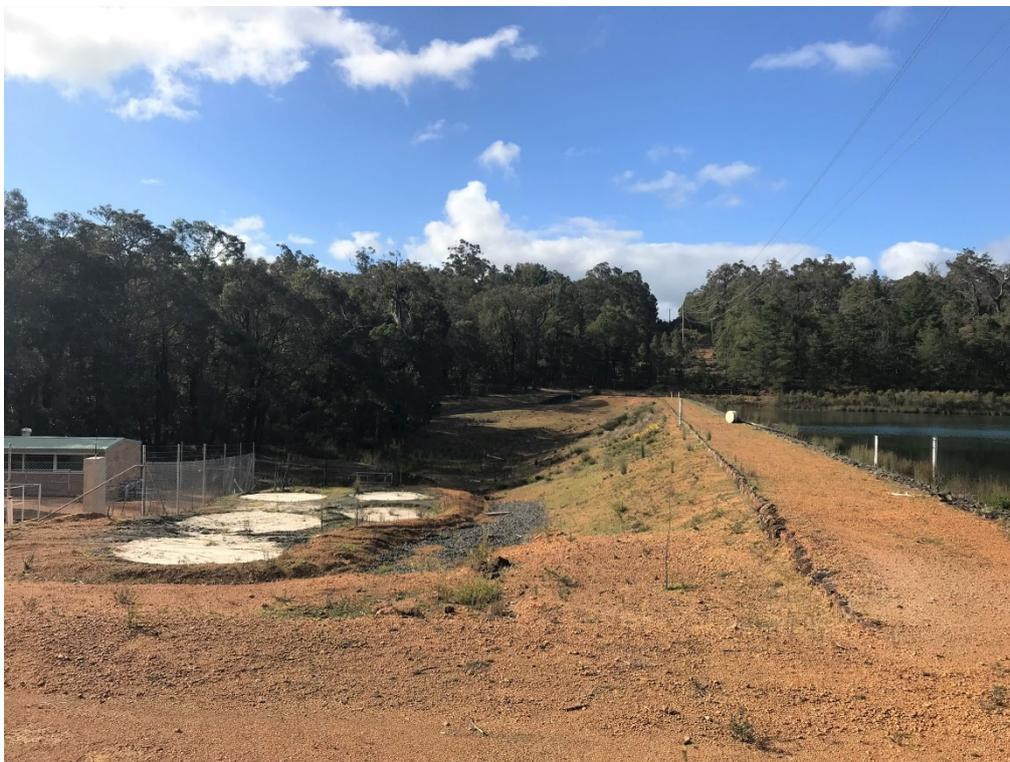
**Figure C4** *Dumpling Gully Dam 1 showing decommissioned water supply tanks due to the source being no longer used by the Water Corporation*
