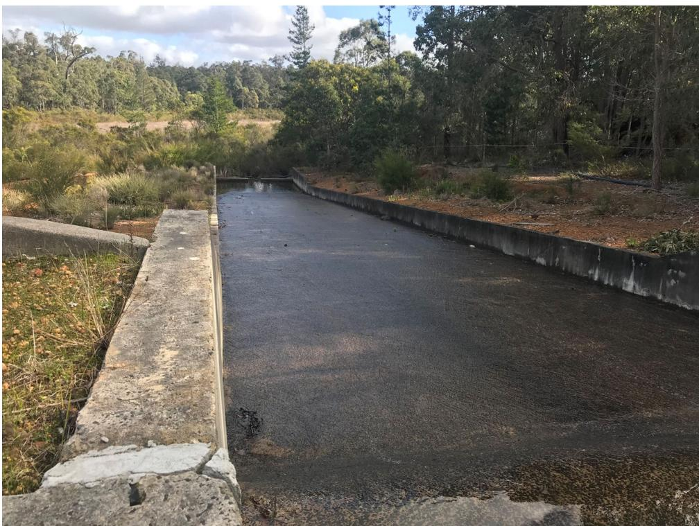
*Figure C2 Spillway from Dumpling Gully Dam 2, overflowing*
