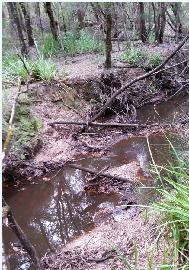
Low water levels in Scotsdale Brook, January 2018. Note the erosion of the banks.
