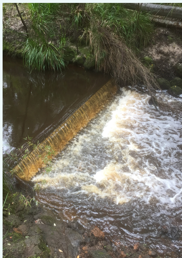
The weir at the Scotsdale Brook sampling site, note the tannin-stained water, July 2018.
