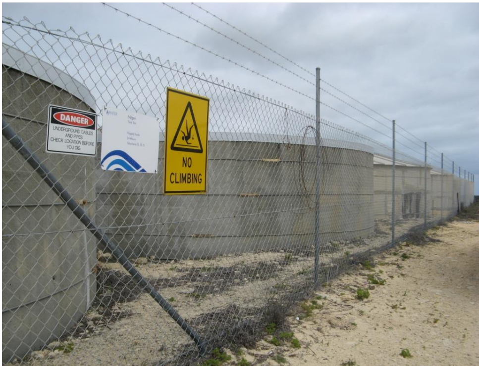
Photograph C4 Nilgen tank site (5 tanks) stores treated drinking water before being gravity fed to residences
