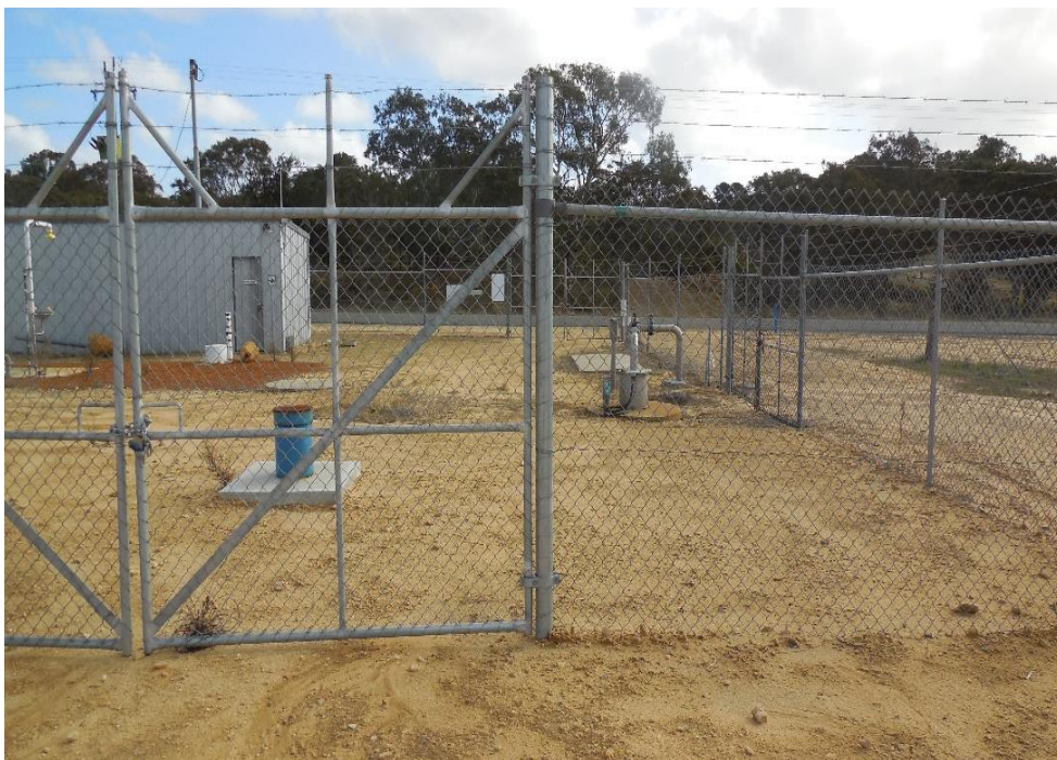
Photograph C2 Bore 1/19 (blue) has been drilled in the same compound as Bore 1 but is not yet equipped to abstract water (looking west)
