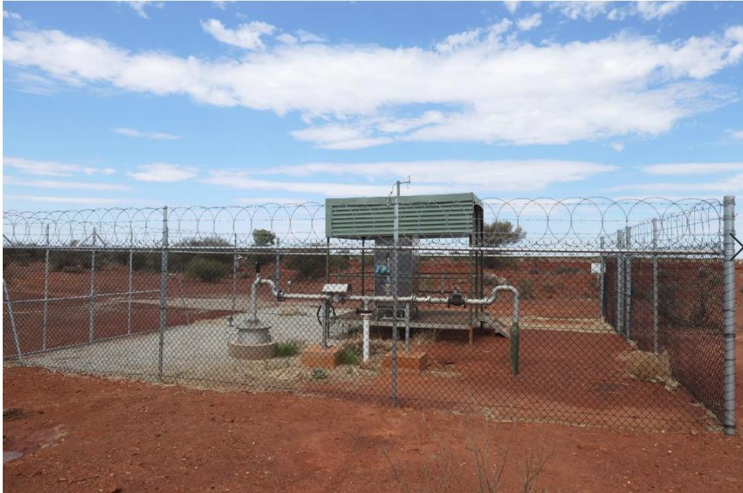
Figure C1 *New production bore 2/16 in a secure fenced compound*
