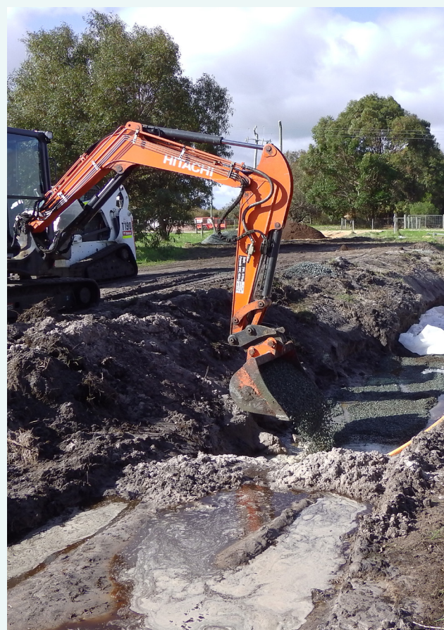
Installing treatment beds in Gull Road Drain that use a high phosphorus-adsorbing material to remove some of the phosphorus from the water, August 2017.
