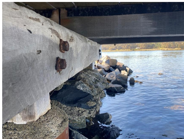
Figure 6. Corroded Bolts
