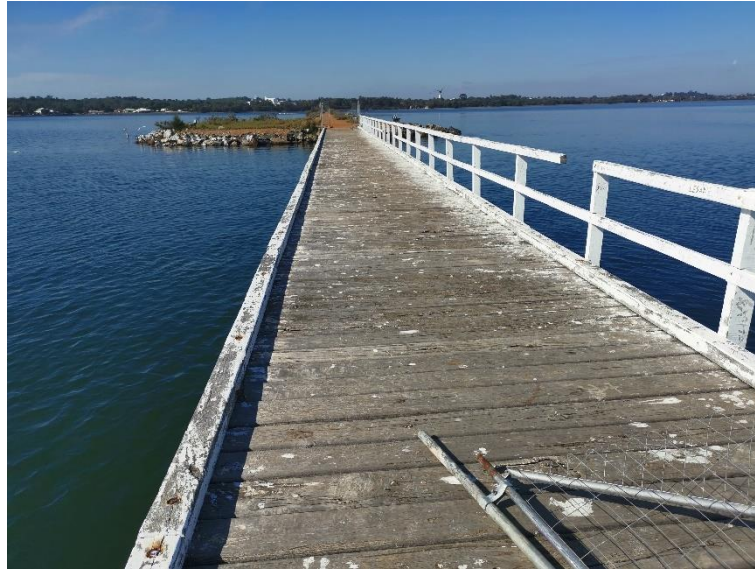
Figure 29. Weathered Deck Board and Broken Handrail
