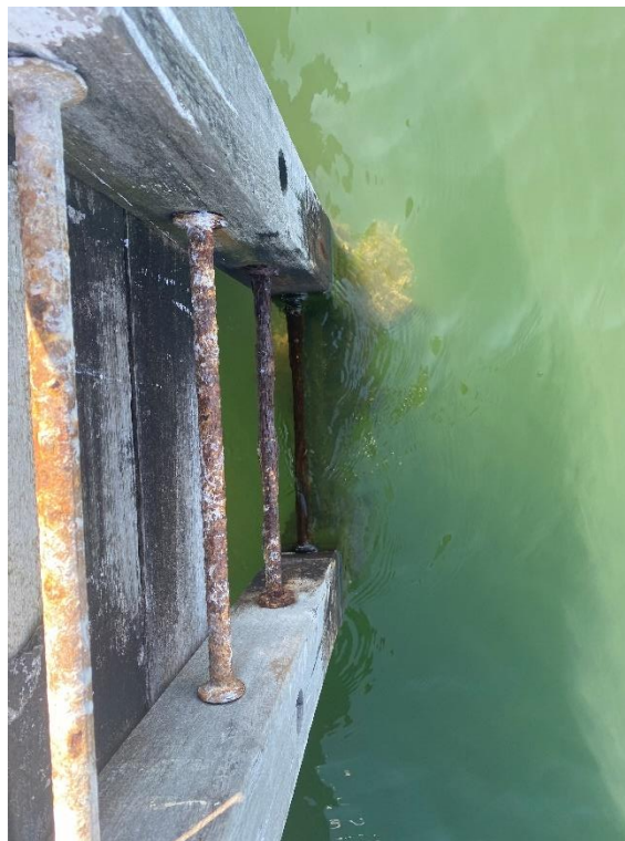
Figure 34. Rusted Ladder
