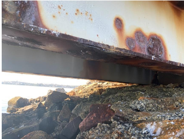
Figure 28. Rusted and Delaminated Steel Beam
