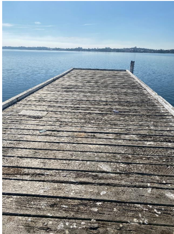
Figure 35. Weathered Deck Board
