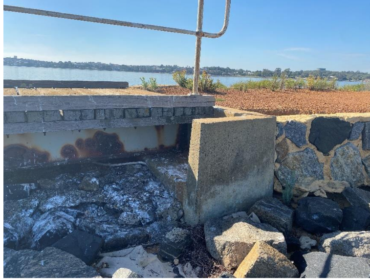
Figure 26. Rusted Steel Beam
