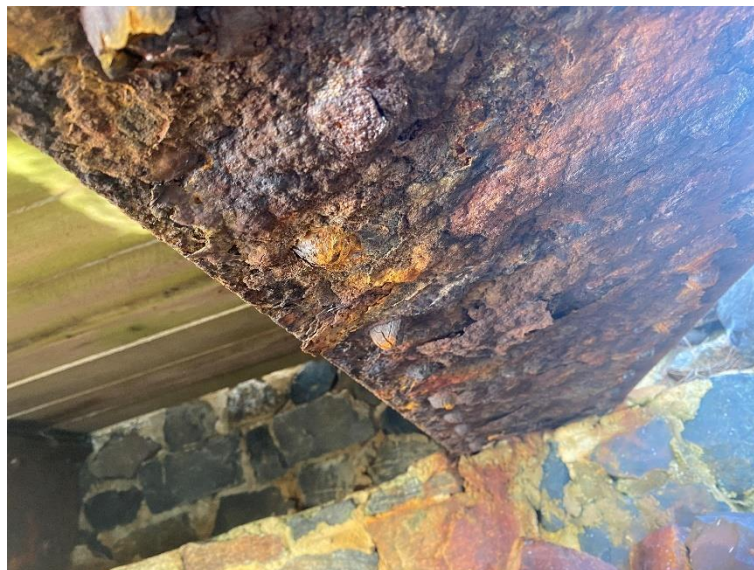
Figure 10. Rusted and Delaminated Steel Beam
