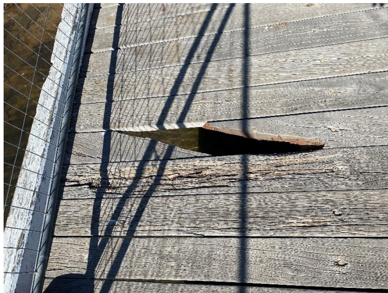
Figure 2. Damaged Deck Board
