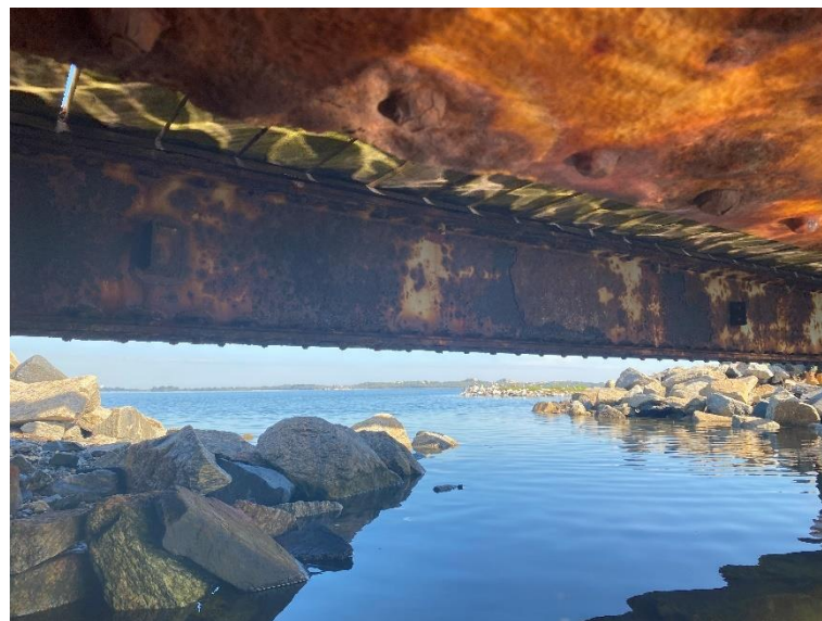
Figure 14. Rusted and Delaminated Steel Beam
