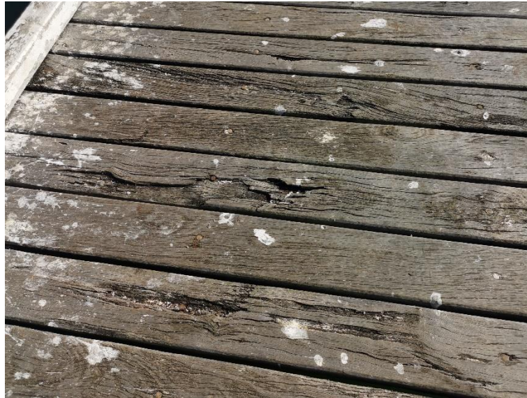
Figure 33. Soft, weathered and Broken Deck Board
