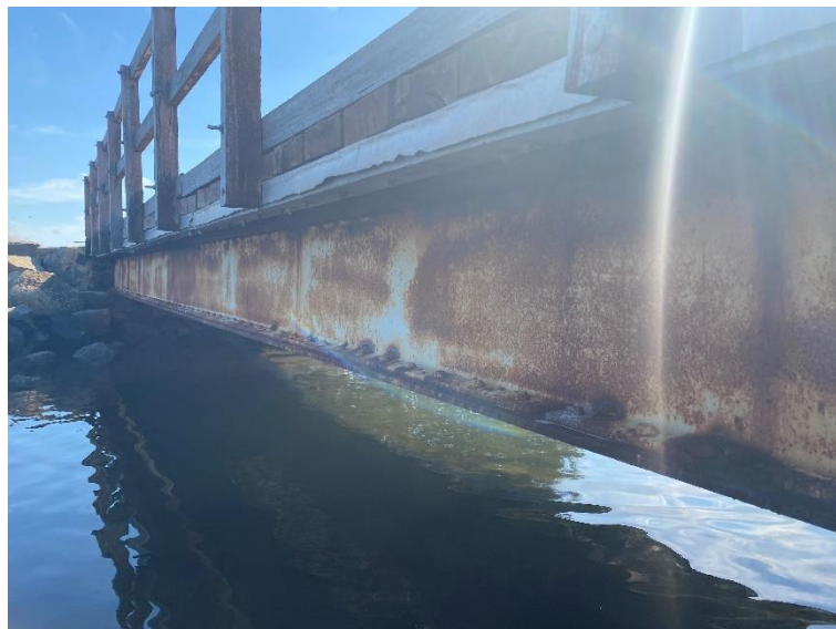
Figure 12. Corroded Steel Beam
