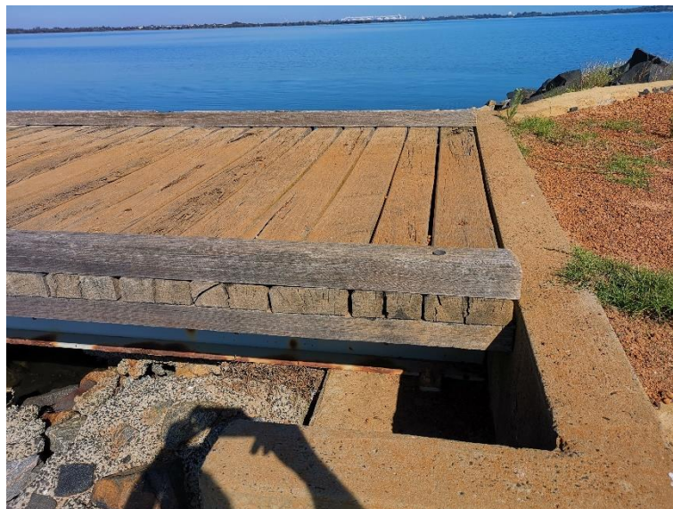
Figure 21. Weathered Deck Board
