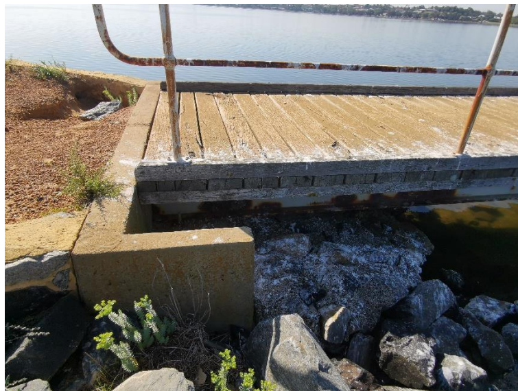
Figure 23. Corroded Handrail, Weathered Deck Board and Abutment
