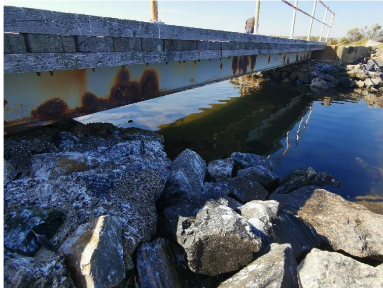
Figure 22. Corroded Steel Beam
