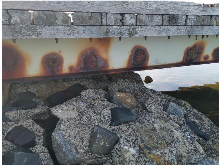
Figure 20. Abutment and Corroded Steel Beam
