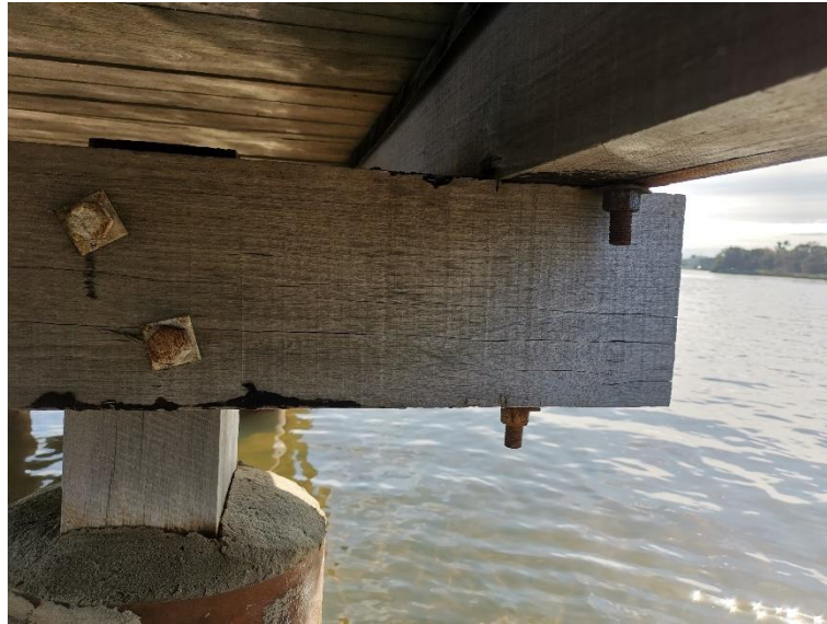
Figure 7. Corroded Bolts
