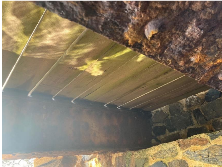
Figure 11. Delaminated and Rusted Steel Beam
