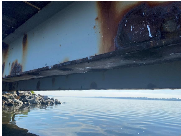
Figure 27. Delaminated Steel Beam
