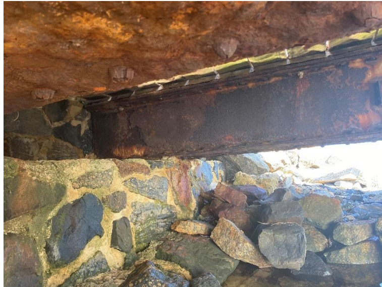
Figure 15. Abutment and Rusted Steel Beam
