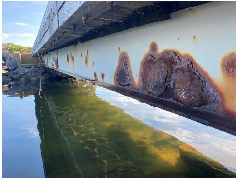
Figure 18. Delaminated Steel Beam
