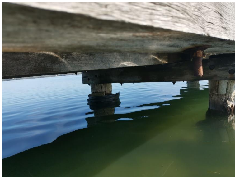
Figure 30. Damaged Encapsulation in Piles
