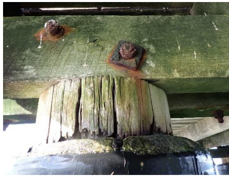
Image 2. Example of Typical Halfcap Connection at each pile
