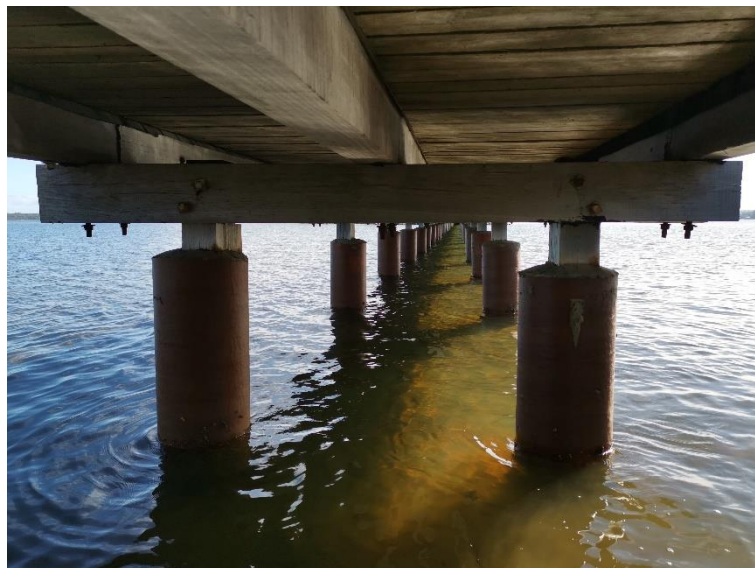
Figure 4. Piles and Corroded Bolts
