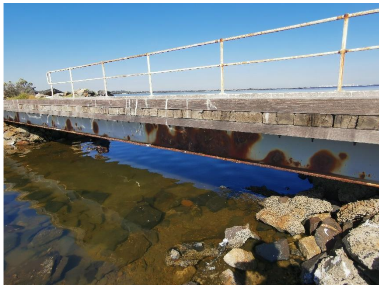
Figure 25. Delaminated and Rusted Steel Beam
