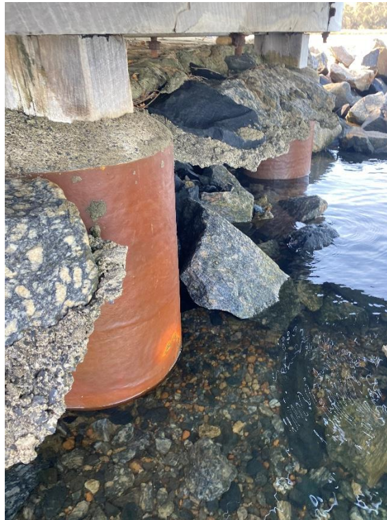
Figure 5. Encapsulated Piles
