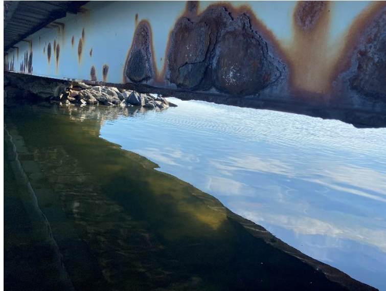
Figure 16. Corroded Steel Beam
