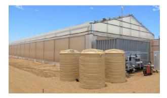
The project was an upgrade/refurbishment of the existing research facility that will allow researchers to examine how the Gravo greenhouse can be used to optimise production of the main vegetables crops that are grown in the district. The roof structure can be open to take full advantage of the sun and shut when there is heat stress, rainfall, high pest pressures and low temperatures to protect the plants.
