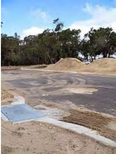
Figure 4. Soil entering a side entry pit that has a soakwell at the base; located within a pipeless subdivision within the City of Mandurah, WA. (Photograph: Department of Water 2007.)
