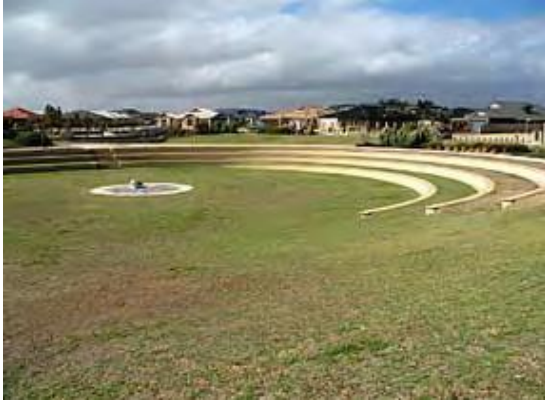
Figure 1. Landscaped POS Infiltration Basin, Quandong Park, City of Mandurah. (Photograph: Department of Water 2007.)
