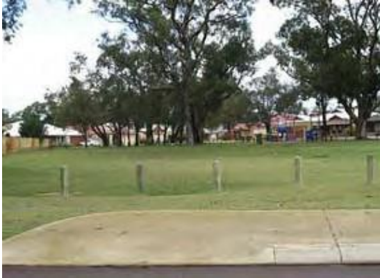
Figure 1. Detention basin retrofit, Bridgewater, City of Mandurah. (Photograph: Department of Water 2007.)
