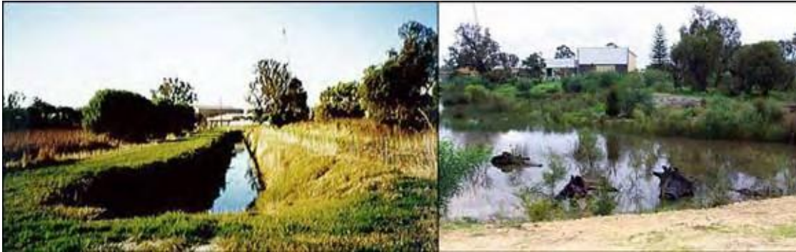
Figure 7. Black Creek trapezoidal drain converted to a constructed wetland, City of Canning. (Photographs: (left) JDA 1999, (right) Water and Rivers Commission 2003.)
