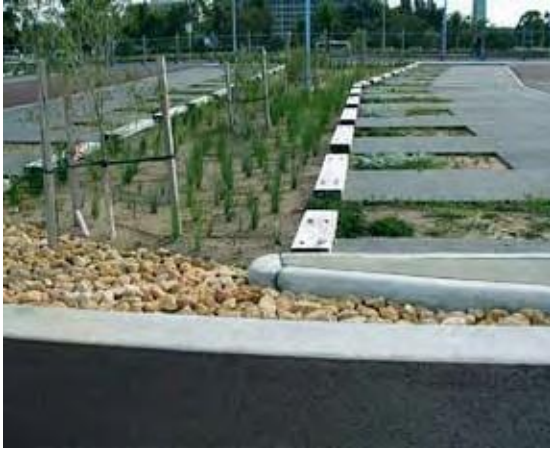
Figure 1. Flush kerbing and broken kerbing used to allow flow from a carpark into a swale at Point Fraser, Perth. (Photograph: Department of Water 2006.)
