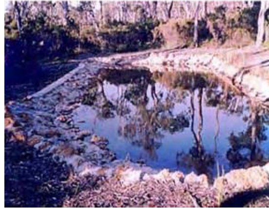
Figure 10. Flow dissipation structure at outlet of subcatchment. (Photograph: TME 2003.)
