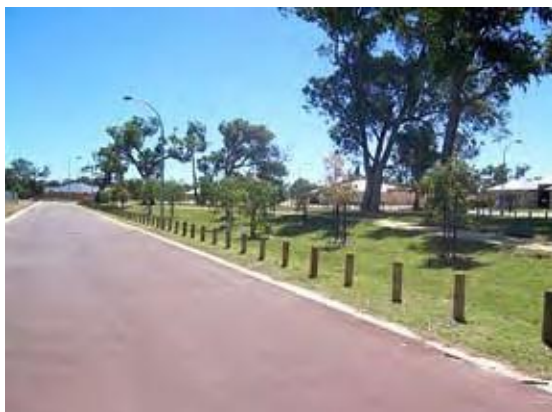
Figure 3. Bollards used to prevent vehicular access onto a swale for conveying road runoff in Mandurah. (Photograph: Grahame Heal, City of Mandurah.)
