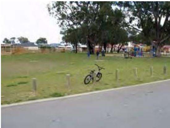
Figure 6. Flush kerbing to allow dispersion of road runoff into adjacent parkland. (Photograph: Department of Water 2006.)
