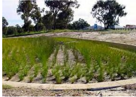
Figure 2. Bioretention area constructed in the Treendale development, Australind. (Photograph: Wayne Edgeloe, Thompson McRobert Edgeloe (TME) Consultants, 2006.)
