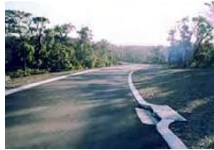
Figure 8. Streetscape of constructed system. (Photograph: TME 2003.)
