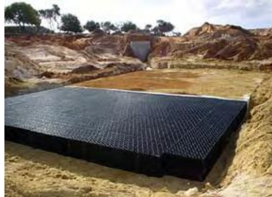
Figure 2. Crate cell infiltration basin system below POS, City of Mandurah. (Photograph: Grahame Heal, City of Mandurah 2004.)
