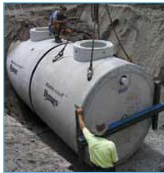
Concrete underground tank
