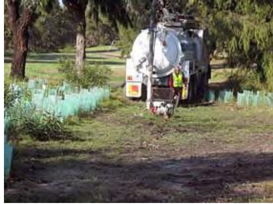
Figure 5. Bubble-up pit located in Bindaree Reserve, Joondalup, being cleaned using a vacuum truck. (Photograph: Department of Water 2006.)
