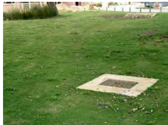
Figure 5. Grassed swale and bubble-up. (Photograph: Department of Water 2006.)
