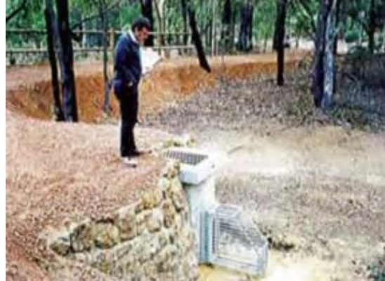
Figure 2. Darkan Street Detention Basin with riser outlet, Shire of Mundaring. (Photograph: JDA 1997.)
