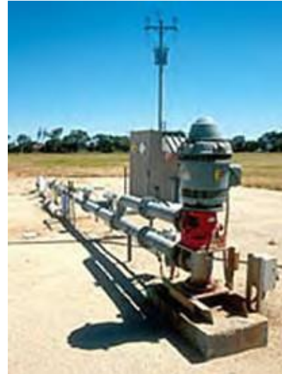
Wastewater aquifer storage and recovery pump at Bolivar, South Australia. (Photograph: CSIRO Land and Water website © CSIRO 2005.)
