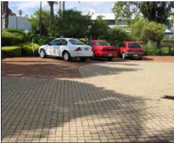
Figure 1. Pervious paving in a commercial carpark, Burswood. (Photograph: Department of Water 2006.)
