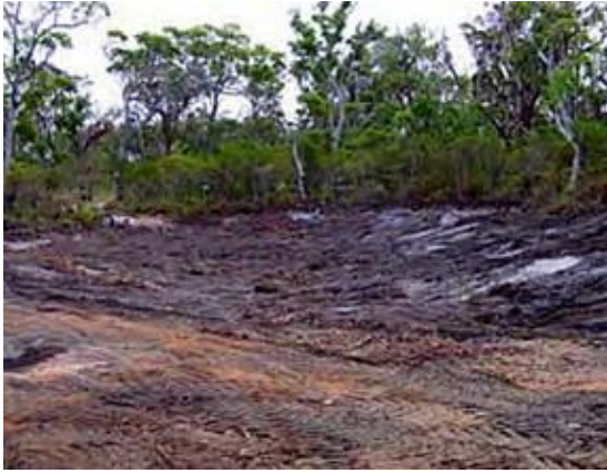
Figure 9. Extended detention basin construction in Stage 2. (Photograph: TME 2003.)
