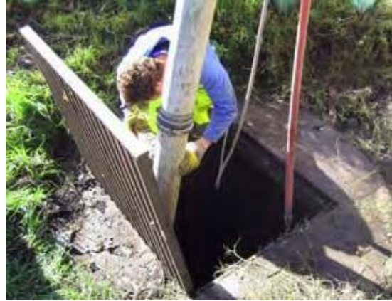
Figure 2. Maintenance of a litter and sediment trap, upstream of Lake Goollelal, Kingsley. (Photograph: Department of Water 2006.)
