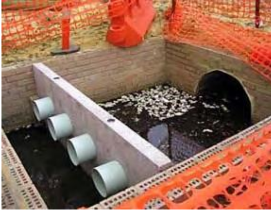
Figure 1. GPT upstream of Liege Street Wetland, Cannington. (Photograph: Department of Water 2004.)
