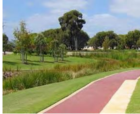
Figure 2. Vegetated swale in Gosnells, making use of native species in a parkland setting. (Photograph: Department of Water 2004.)
