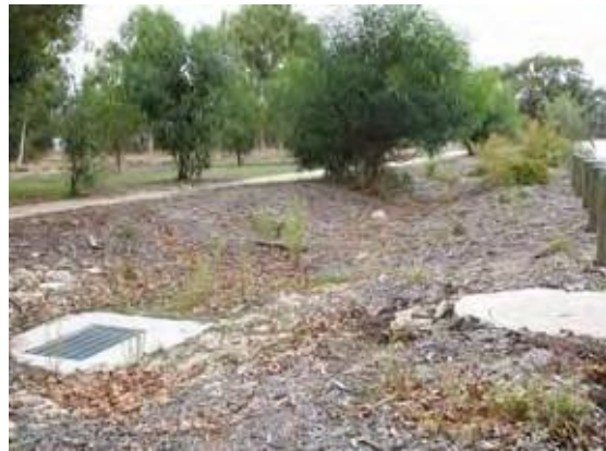
Figure 7. Bubble-up pit located within a swale at the downstream end of the catchment. (Photograph: Department of Water 2007.)
