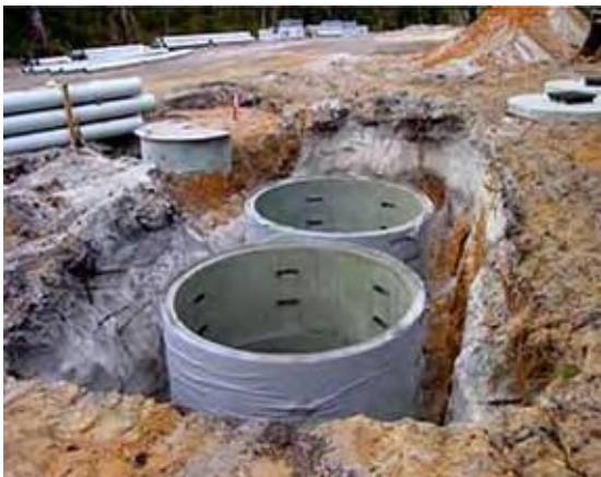
Figure 5. Soakwell construction. (Photograph: TME 2003.)
