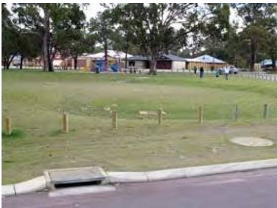
Figure 4. A multiple use park incorporating a landscaped stormwater detention area. (Photograph: Department of Water 2006.)
