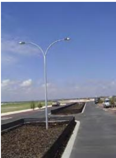
Figure 4. Newly constructed and mulched swale. (Photograph: Ardross Developments 2004.)
