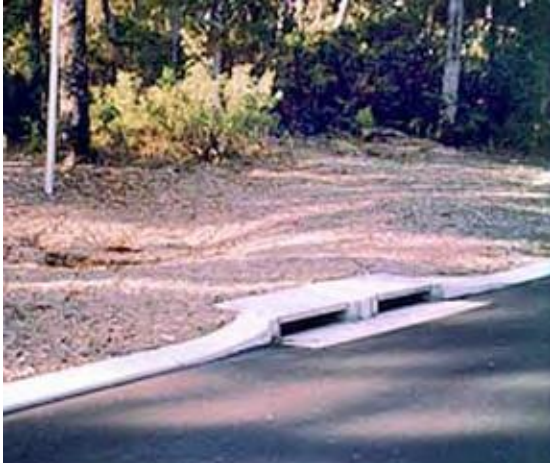
Figure 3. Side entry pit and bubble-up located within mulched detention area. (Photograph: TME 2003.)
