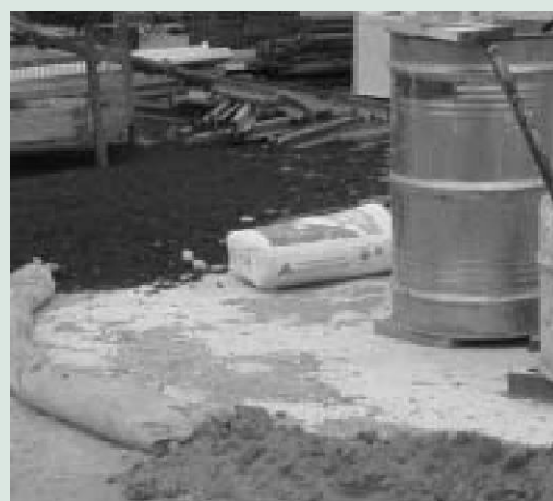
Figure 4. Contained wash area to collect runoff. (Photograph: Clean Site, Keep Australia Beautiful Council WA.)
