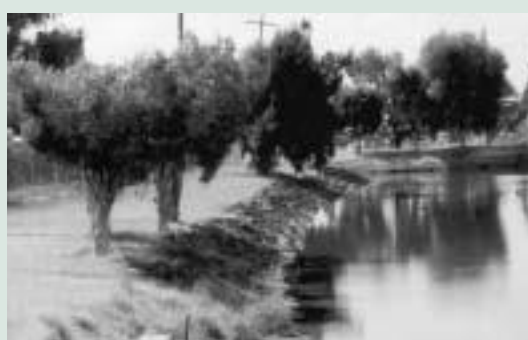
Figure 9. Sediment cleared from a stormwater compensation basin and spread on the banks. Mill Street Compensation Basin, Welshpool. (Photograph: Department of Environment.)
