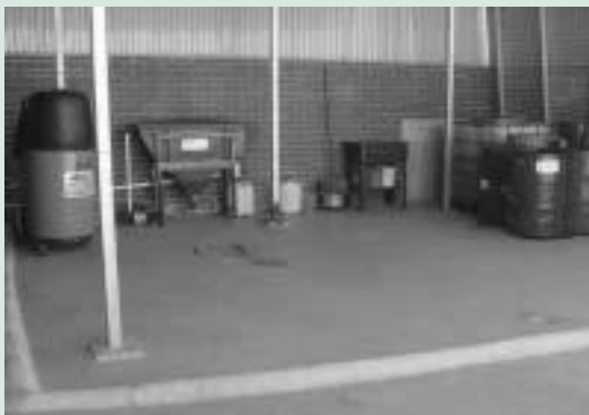
Figure 15. Green Stamp automotive premises, Balcatta. Undercover, bunded, wash-down area, with parts washer, wastewater treatment equipment and drums for recyclable materials. (Photograph: Department of Environment.)
