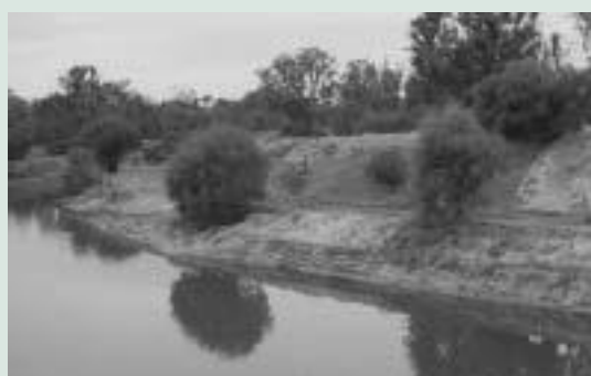
Figure 8. Sediment excavated from the Harvey Main Drain and stockpiled on the banks. Sediment has buried fringing vegetation and may be washed into the waterway. (Photograph: Department of
