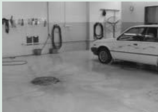
Figure 16. Green Stamp automotive premises, Balcatta. Vehicle wash-down area, with collection drain for wastewater treatment. (Photograph: Department of Environment.)
