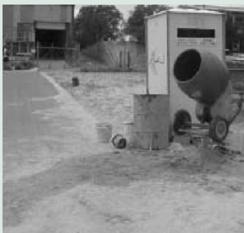
Figure 3. Cement mixer wash-water runoff and sand on the road. (Photograph: Clean Site, Keep Australia Beautiful Council WA.)
