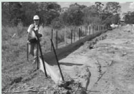
Figure 7. Silt fence for controlling sediment during land development. (Photograph: André Taylor, Ecological Engineering Pty Ltd.)
