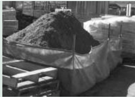
Figure 6. Soil stockpile contained by a sediment fence. (Photograph: Clean Site, Keep Australia Beautiful Council WA.)
