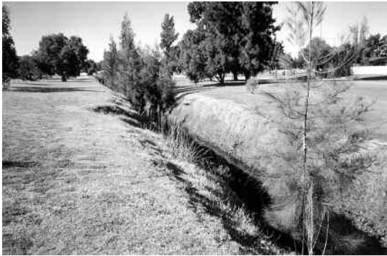
Figure 29: Bannister Creek before restoration works (1999) – a straight trapezoidal drain with steep grassed banks and high velocity flows. (Photograph: former Department of Environment)
