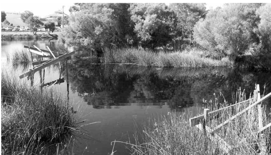
Figure 27: Straight drain converted to a vegetated compensating basin, Russell Street, Morley. (Photograph: Debbie Besch, NMCG)
