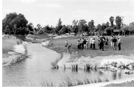
Figure 30: Bannister Creek post-engineering (restoration) works summer 2001. The channel was realigned to create a winding creek and the banks reshaped to a gentle slope and stabilised. (Photograph: former Department of Environment)
