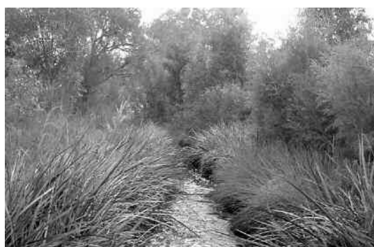
Figure 32: Bannister Creek 2004. Revegetation was undertaken to reduce water velocity, control erosion and rehabilitate the drain into a living stream. Flooding resulted in no significant damage to the creek. (Photograph: Georgia Davies, BCCG)
