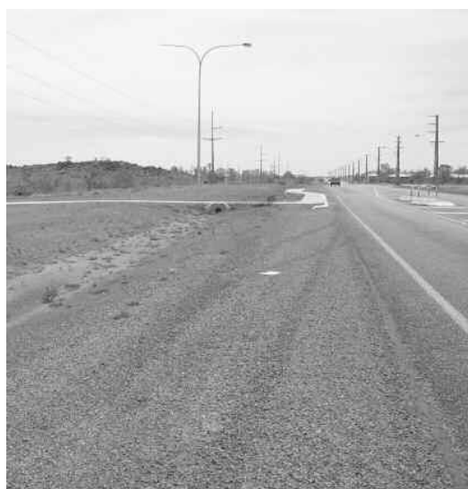
Figure 10: Example of a kerbless road and swale, Dampier Road, Karratha. (Photograph: Department of Environment, 2006)
