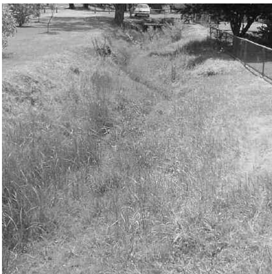
Figure 14: Geegelup Brook, Bridgetown, before restoration works – a weed infested trapezoidal drain. (Photograph: Department of Environment, 2003)
