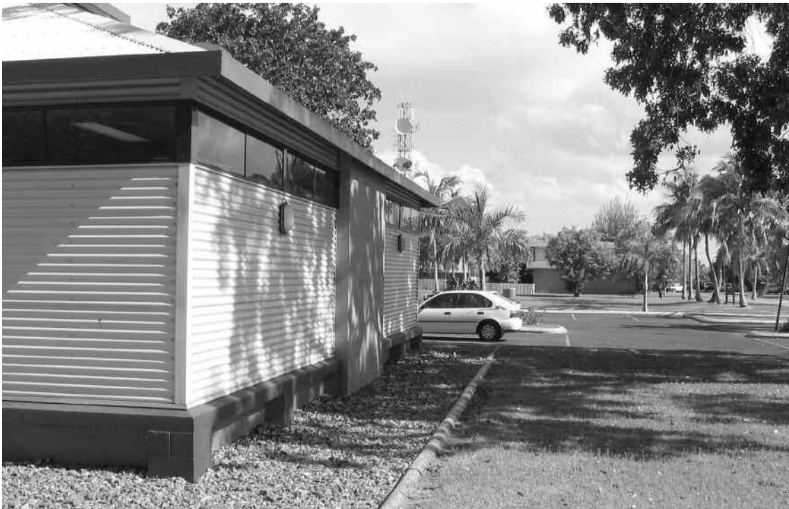
Figure 7: Pervious surface underneath a gutterless roof, Shire of Broome offices, Broome. (Photograph: Allan Ralph, Shire of Broome, 2005.)
