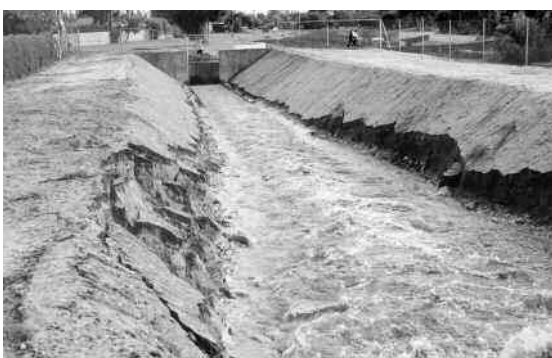
Figure 31: Flood damage of the trapezoidal drain upstream of the rehabilitation reach of Bannister Creek. (Photograph: former Department of Environment)
