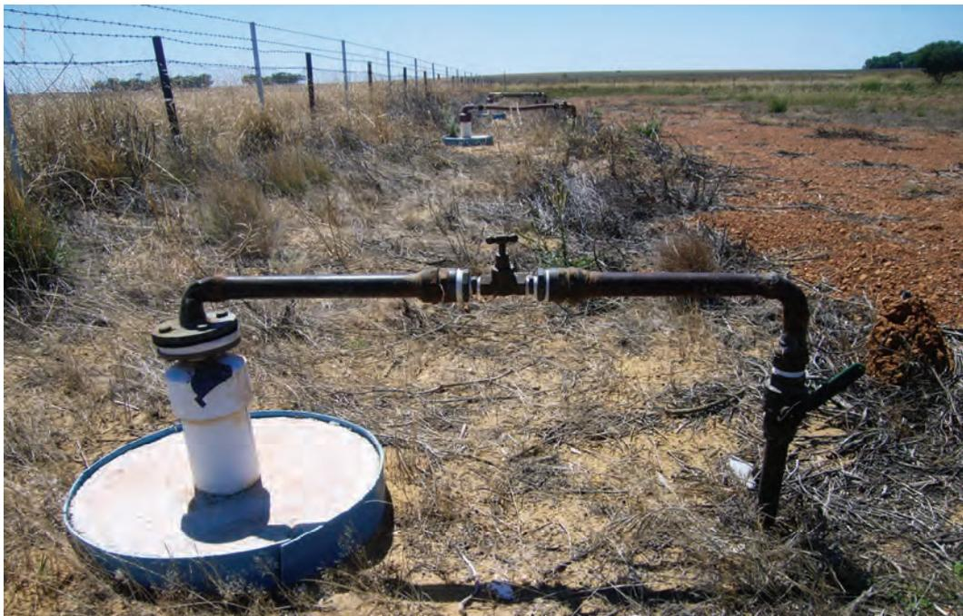
*Figure D2 Capped spears in the Yerecoin well field*
