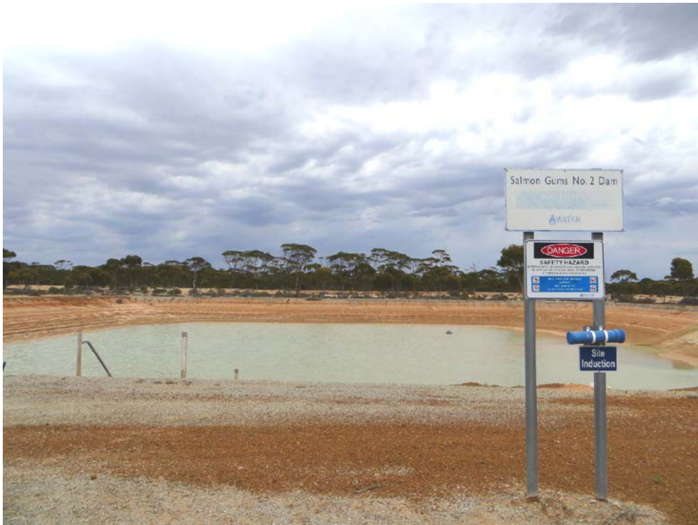
Figure D1 Salmon Gums Dam no. 2, photograph by V. Claughton
