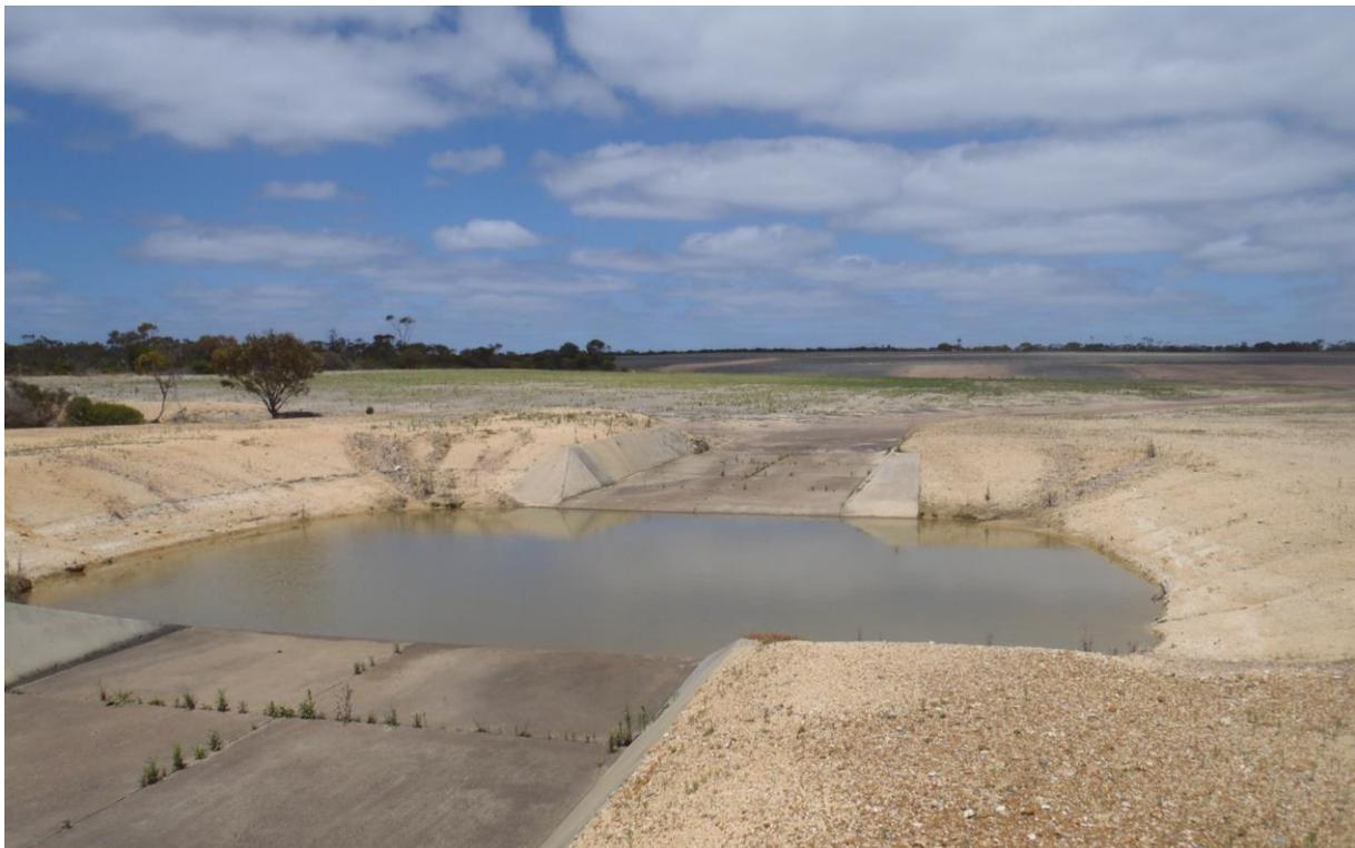
*Figure C2 Sediment trap between the No. 4 dam and the bitumen catchment area*
