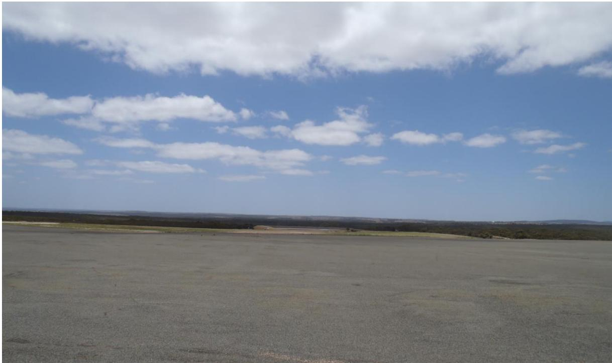
*Figure C1 Bitumen catchment area for the No. 4 dam*
