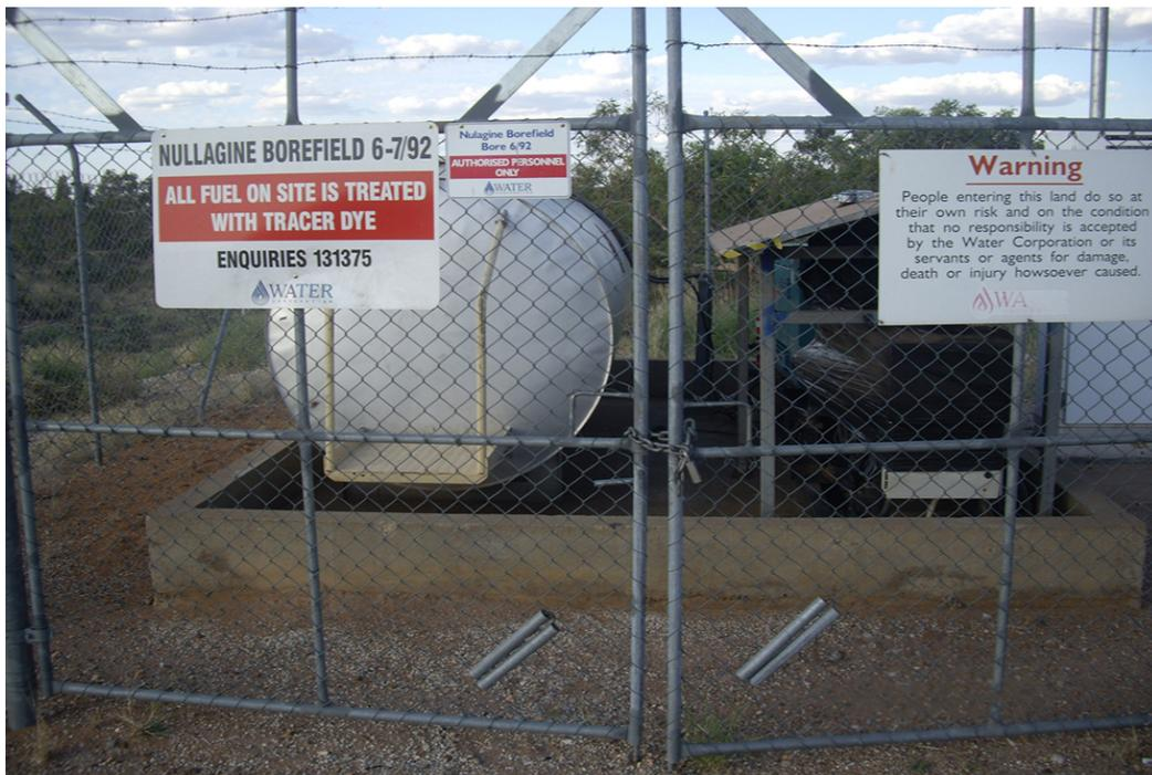
*Figure C3 Diesel storage at a Nullagine Water Reserve drinking water bore site, photograph by N. Mantle, Department of Water and Environmental Regulation*
